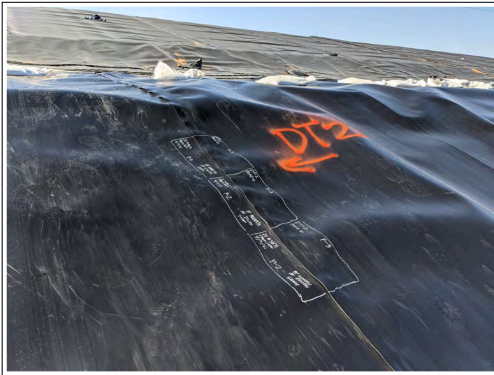
22. 4/7/2021: DT-2 of Pond 6, located on seam P-3/P-2 (view to south)
