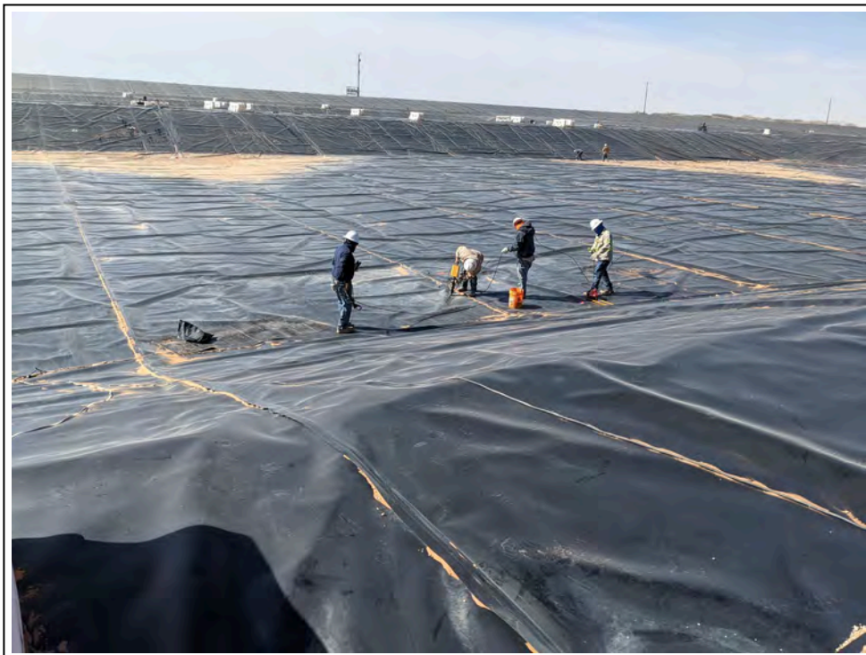
3. 3/31/2021: Crew repairing existing liner in Pond 5; vacuum test was performed on each repair bead and patch (view to southwest)
