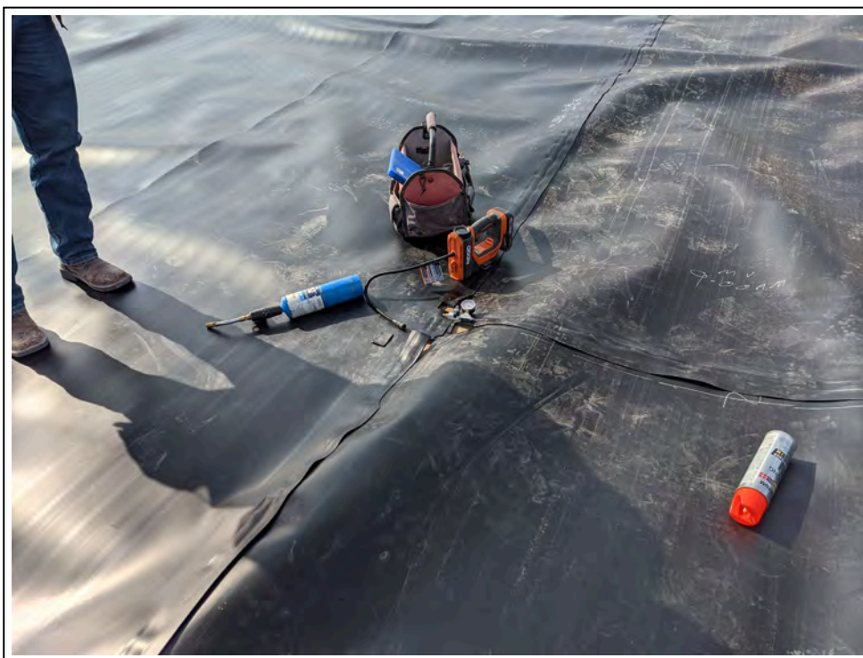
14. 4/2/2021: Seam pressure testing
