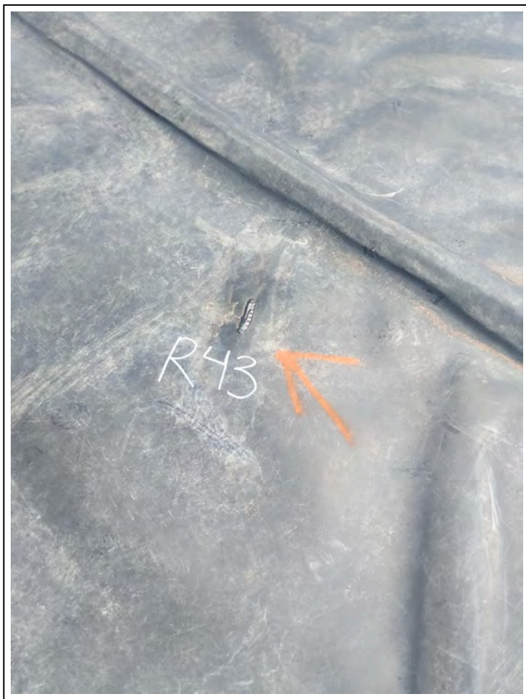
9. 4/1/2021: Pond 5 existing liner repair (bead)
