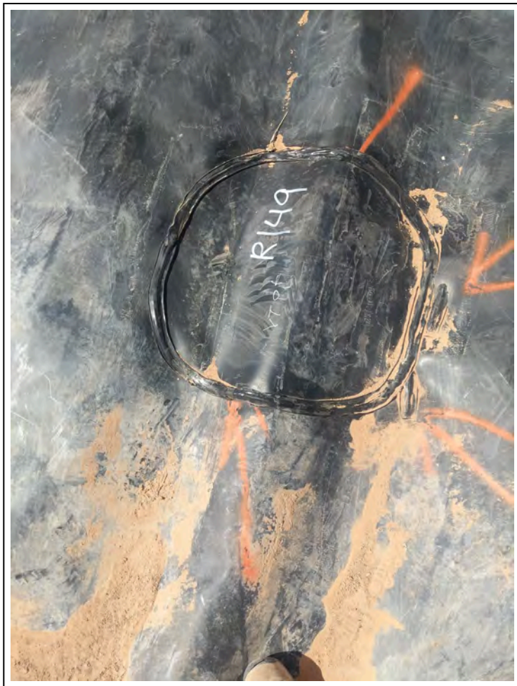
11. 4/1/2021: Pond 6 existing liner repair (patch)
