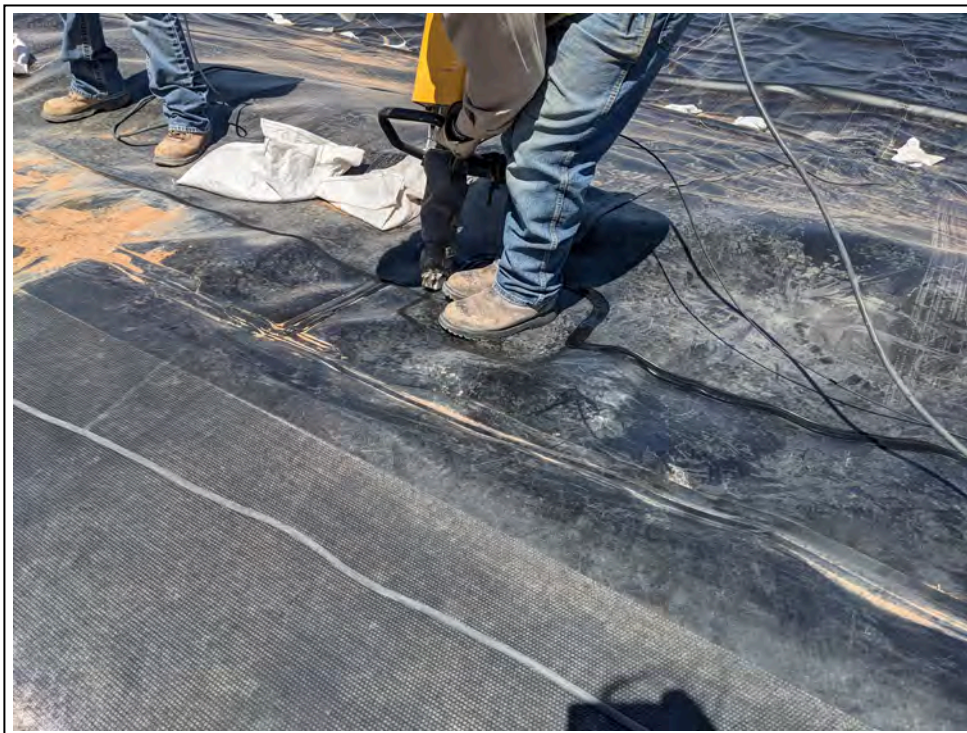
7. 4/1/2021: Top seams extrusion welded; T-seams patched
