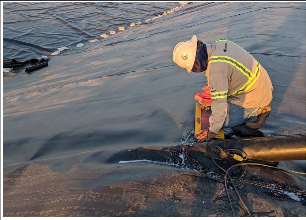
25. 4/9/2021: Vacuum test along northeast extrusion weld seam (view to west)
