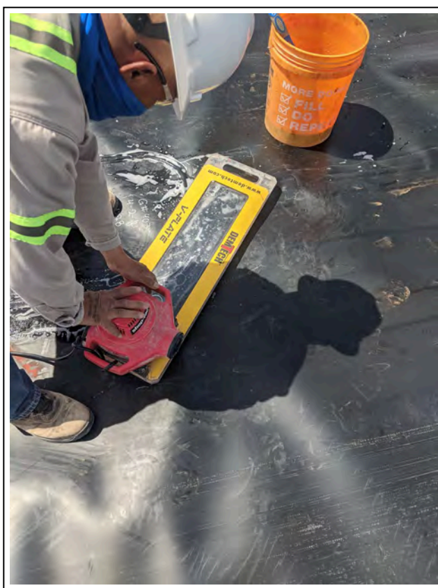
16. 4/2/2021: Vacuum test at DT repair location
