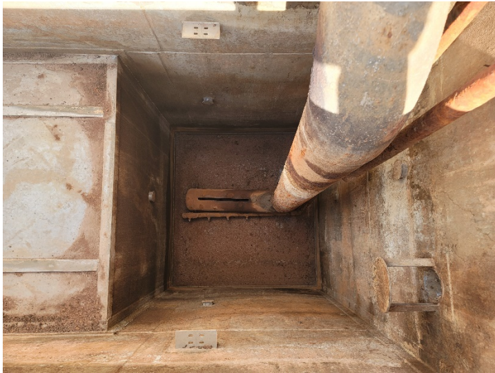
Photo 1. API – East Bay, South End
