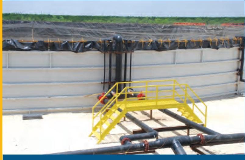
Example of safety clamps on Tank Tech Model 600 tank.
