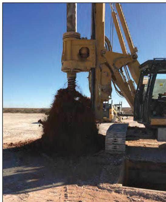
Over the next 2.75 hours the boring was advanced to a total depth of 120 feet with no issue. I inspected the cuttings from each trip for moisture to indicate a groundwater formation and all samples were dry. If any appreciable moisture would have been indicated, the operation would have been suspended to allow the water to accumulate and then measured.
