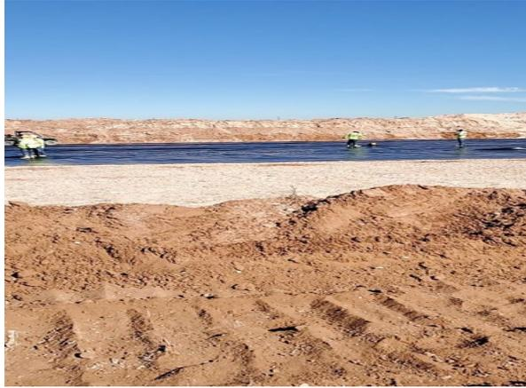
Photo 1: View of liner installation.
