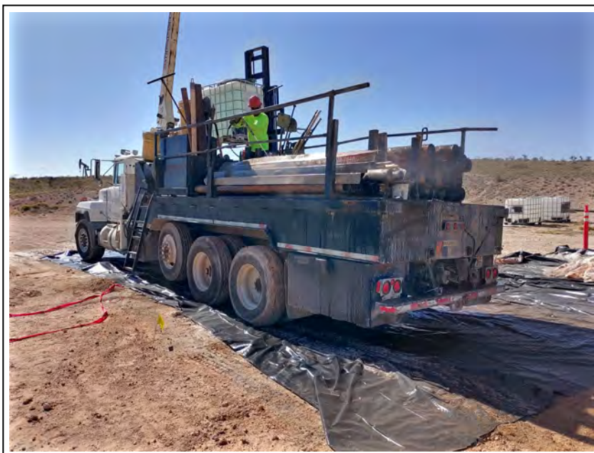
4. Rig decontamination
