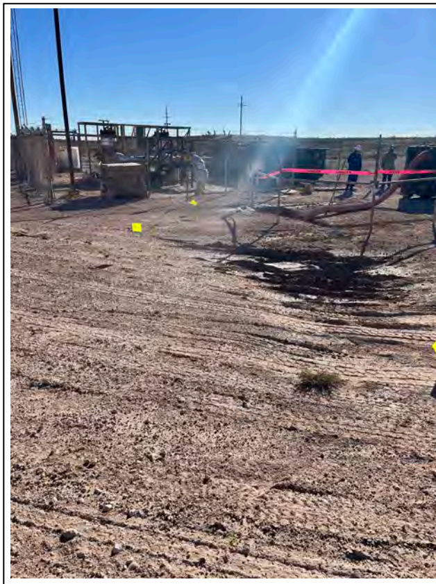
1. Hydrovac excavation at WDW-3-BH-1
