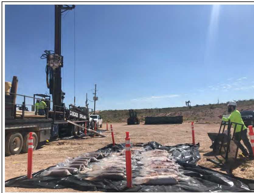
2. Sonic drilling at WDW-3-BH-1, October 5, 2023
