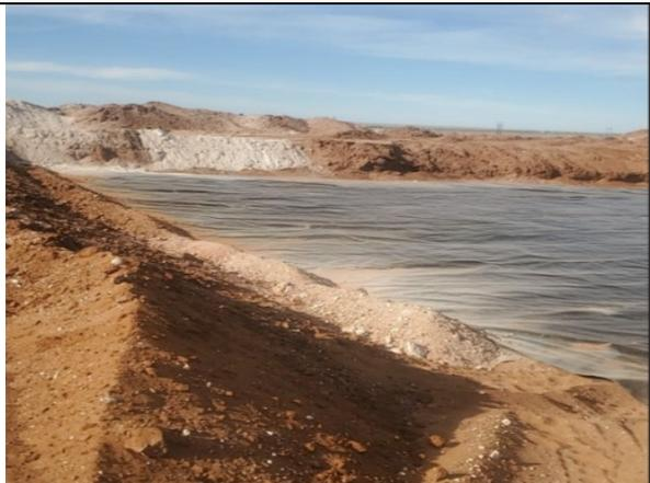
Photo 3: Overview of liner installation.
