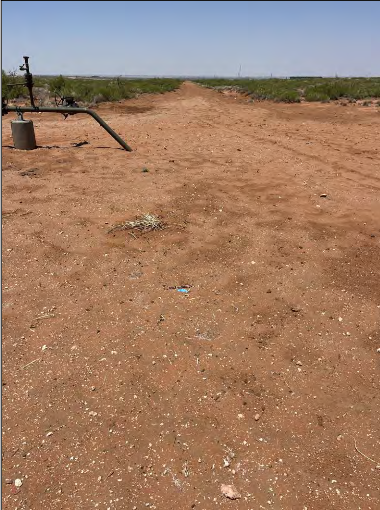
Figure 4: View north-northwest from center of southern boundary of Containment location, identified as location 4. Gas ROW runs NW-SE through western half of Containment location.
