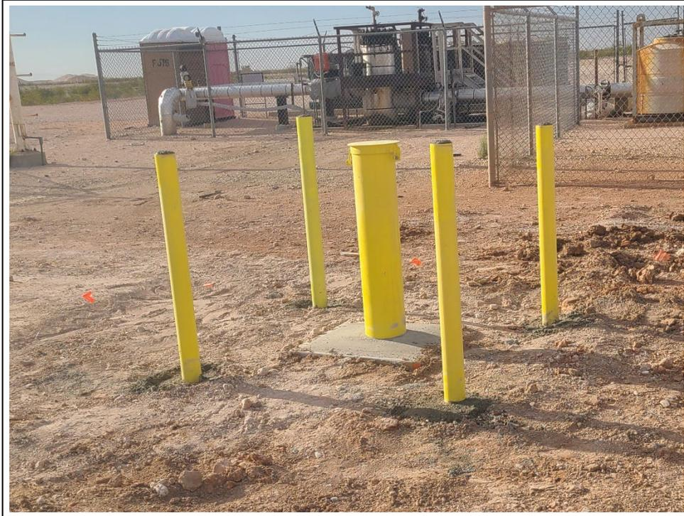
11. 4/28/2025: Well casing and bollards cemented
