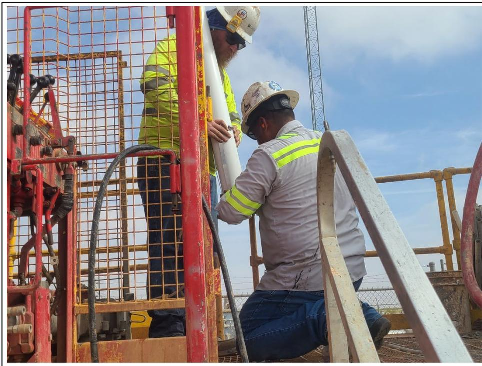
10. 4/24/2025: Cascade setting centralizers on well casing
