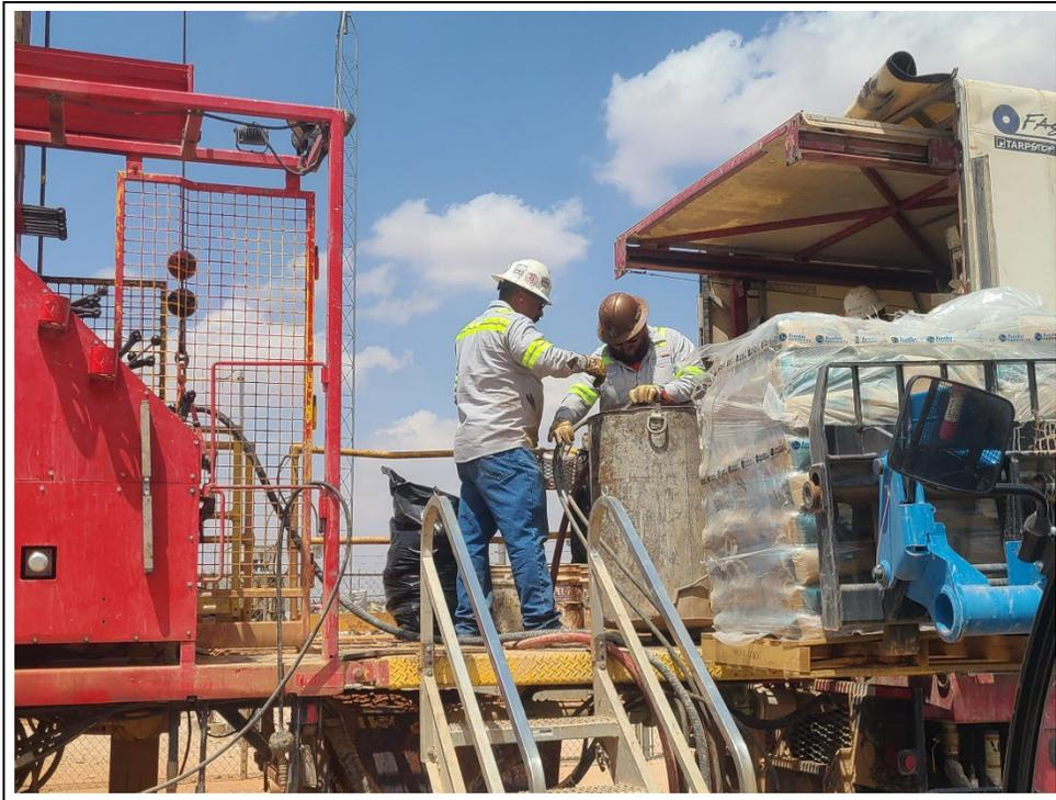
8. 4/26/2025: Cementing from total depth of 500 feet bgs to 325 feet bgs
