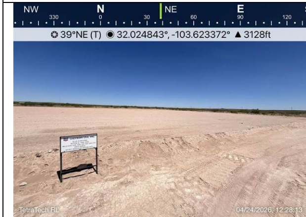
Photo 3: Overview of backfilled pit and pit sign.
