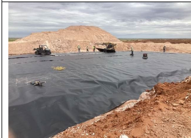
Photo 5: Overview of liner installation at the Salado Draw Pad 366 Pit
