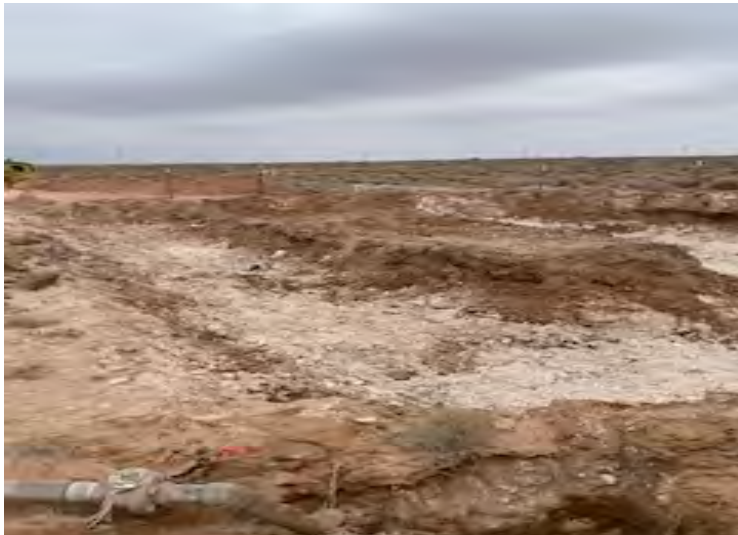
Photograph 3: View of excavation north of point of release
