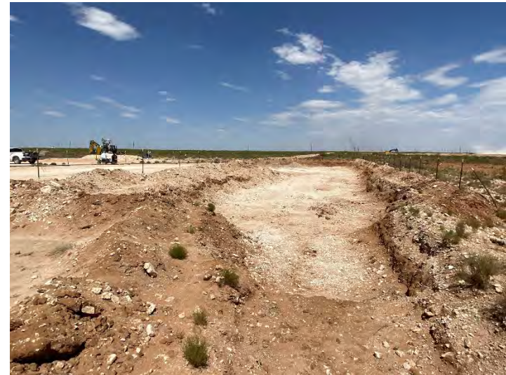
Photograph 8: Eastern view of excavation.
