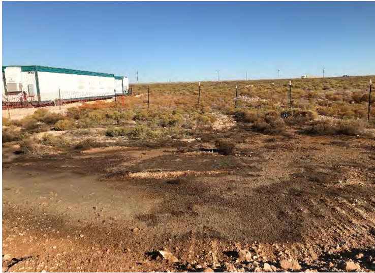
Photograph 1: View of release extent north of point of release.
