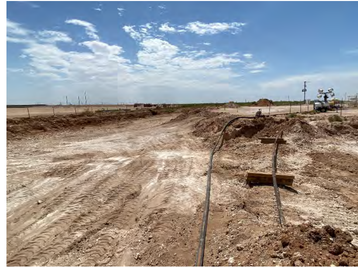
Photograph 6: Western view of excavation.
