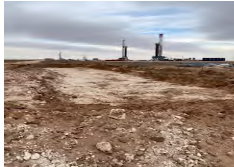
Photograph 4: View of excavation south and west of point of release, facing east.
