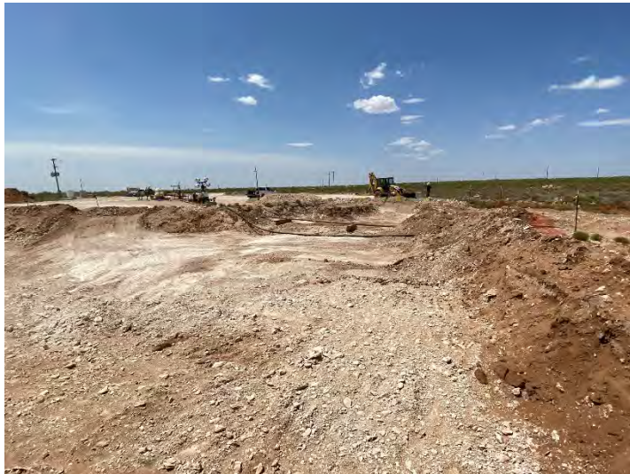
Photograph 7: Northern view of excavation.
