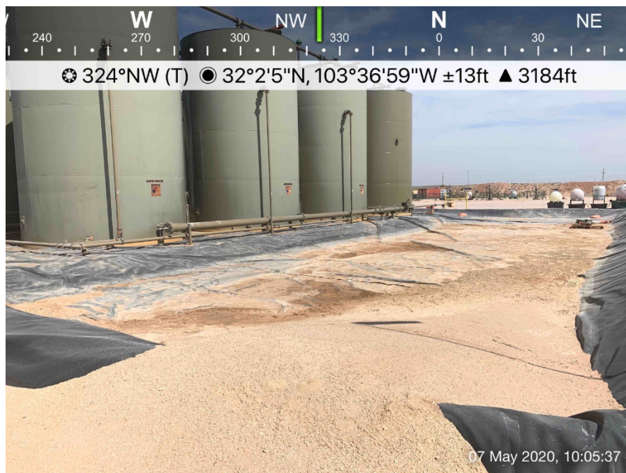
Spill area where release was contained within the lined berm viewing northwest
