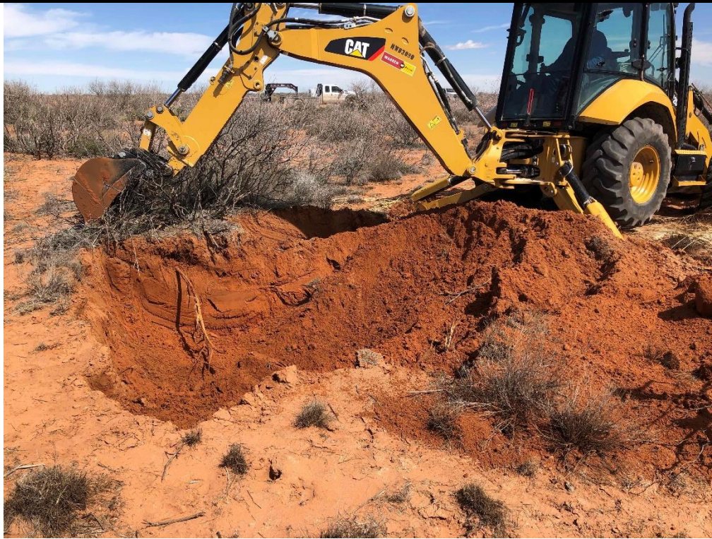
PHOTO 19: View of remediation around HA-5. 6/4/19
