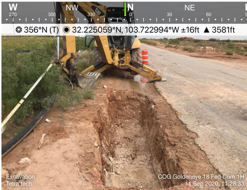
View North, area of Bottomhole 11
