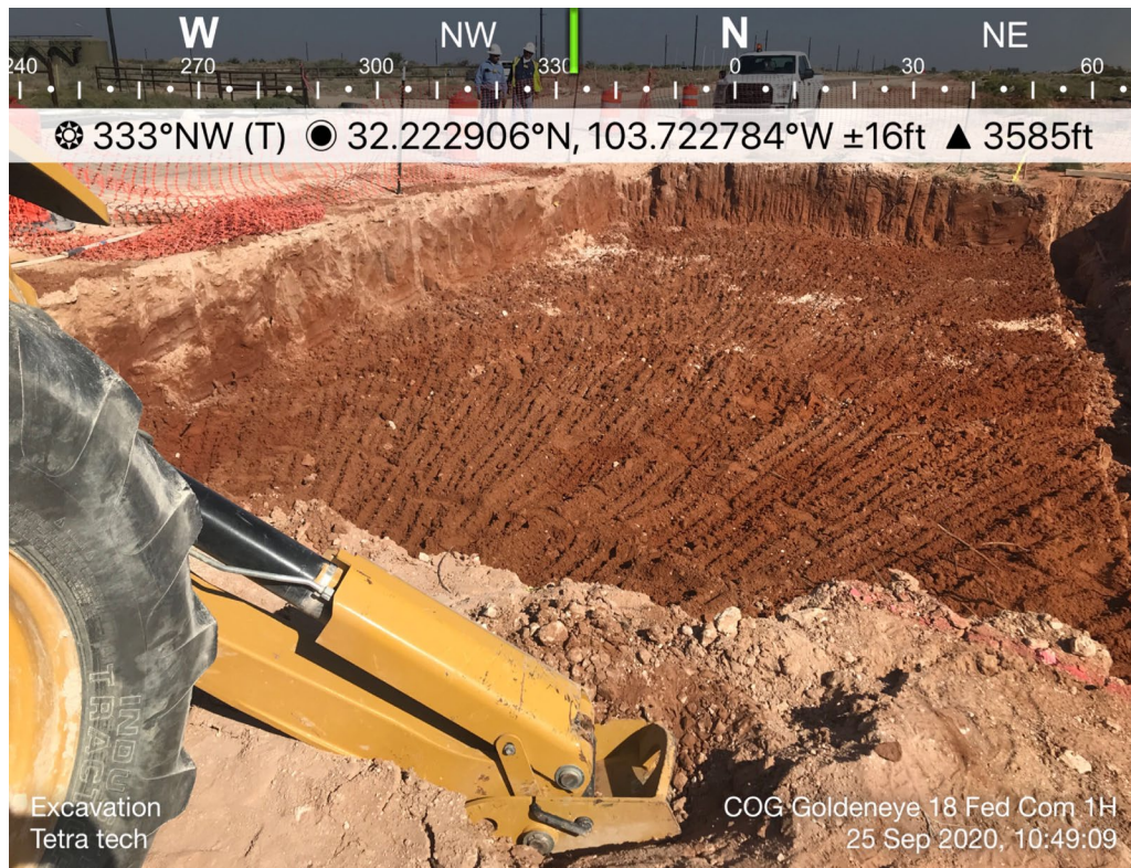
View North, area of Bottomholes 37, 40, 43, and 46
