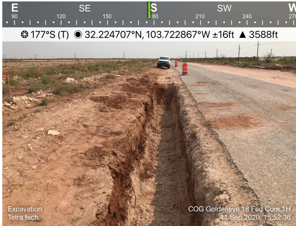
View South, area of Bottomholes 12 and 13
