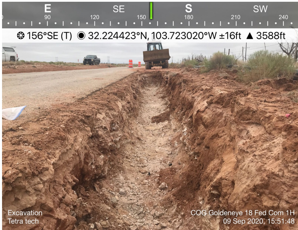
View South, area of Bottomholes 7 and 8
