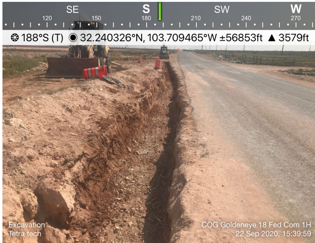
View South, area of Bottomholes 33 through 36
