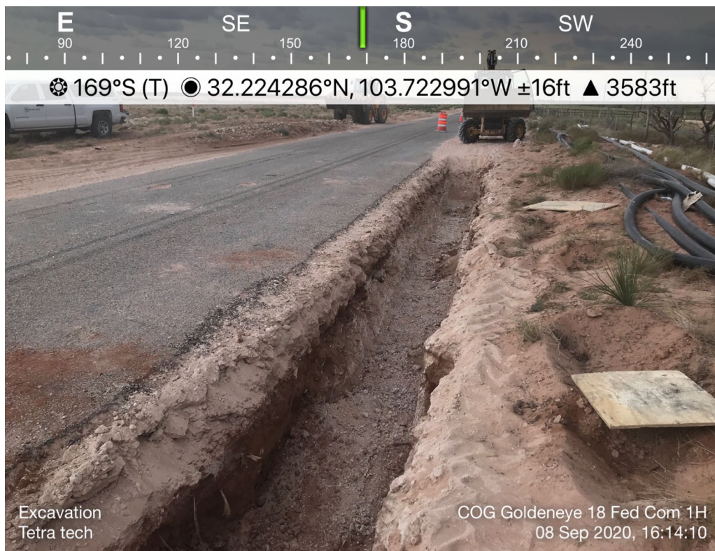
View South, area of Bottomholes 4 through 6
