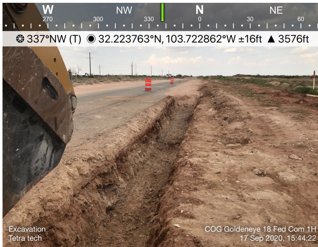
View North, area of Bottomholes 18 and 19
