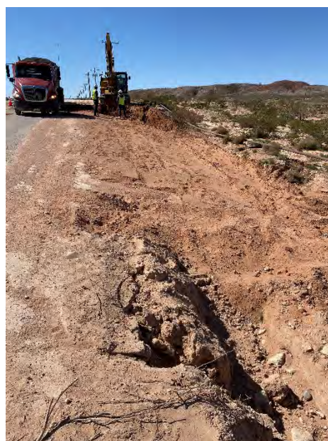
Photograph 4: Southern view of backfilled excavation adjacent to Rawhide Road.
