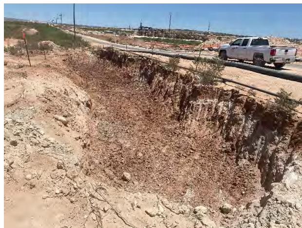
Photograph 6: Northern view of excavation in the pasture adjacent to steel gas flowline.
