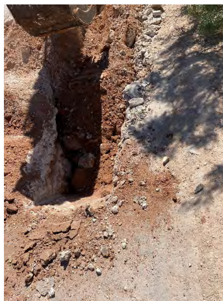
Photograph 8: Caliche observed in a pothole advanced in the lease road at PH05.
