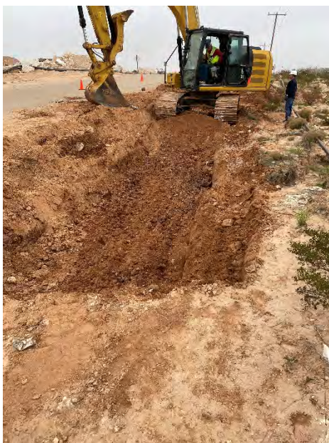
Photograph 3: Southern view of excavation adjacent to Rawhide Road.
