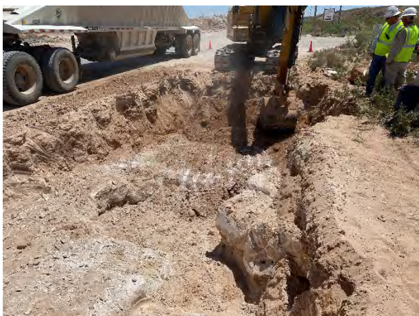
Photograph 5: Southern view of bedrock and boulders in excavation adjacent to Rawhide Road.
