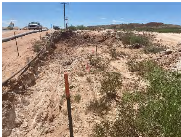
Photograph 7: Southern view of excavation in the pasture adjacent to steel gas flowline.
