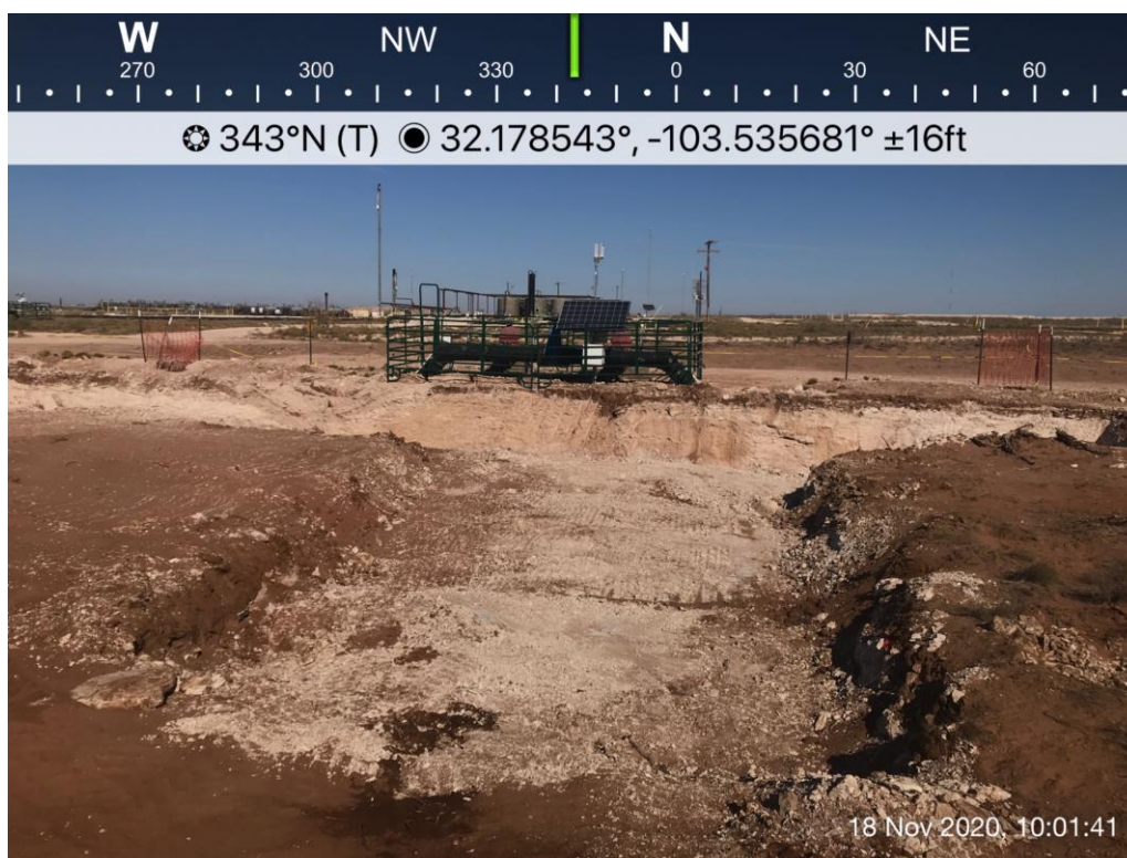
View North, areas of Bottom Holes (9-10)
