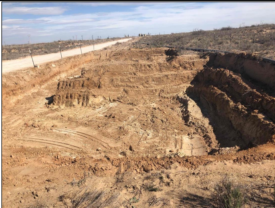
PHOTO 14: View of south of lease road excavation, facing east. 02/03/2020 / TIME: 4:16PM / GPS: 32.6085 -103.4924
