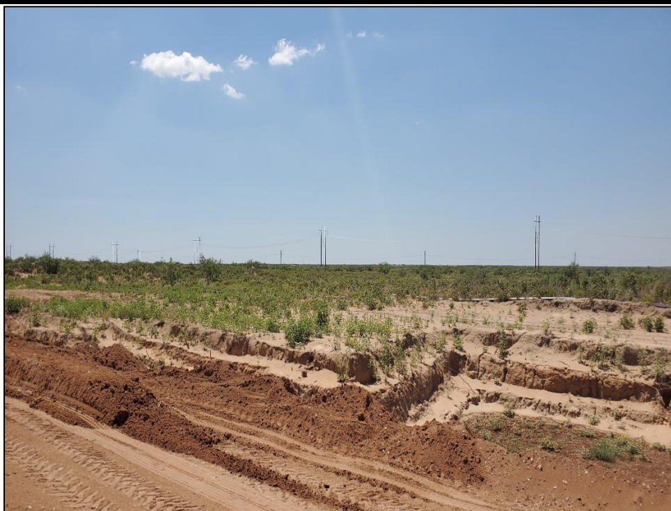
PHOTO 21: View of remediation on lease road. 07/07/2020 / TIME: 11:35PM / GPS: 32.6085 -103.4925
