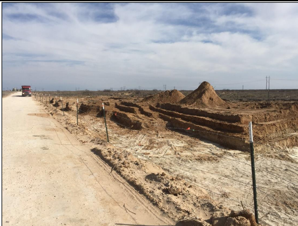
PHOTO 17: View of excavation on the south of lease road. 02/03/2019 / TIME: 3:52PM / GPS: 32.6085 -103.4925
