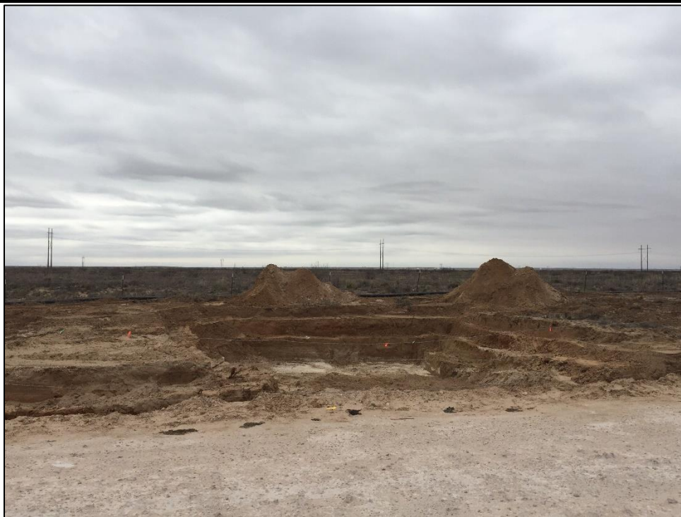
PHOTO 13: View of HA-3, HA-9, GP-2, excavation, facing southwest. 02/19/2020 / TIME: 2:08PM / GPS: 32.6085 -103.4924
