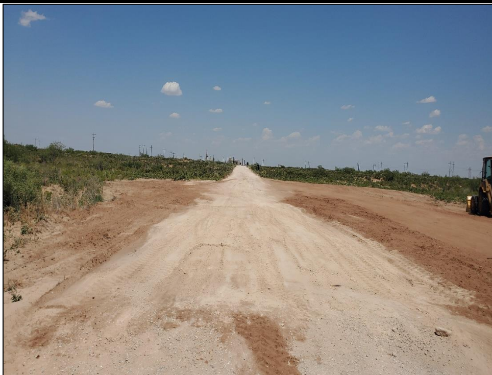
PHOTO 22: View of backfilled excavation from lease road. 07/08/2020 / TIME: 11:35PM / GPS: 32.6085 -103.4925
