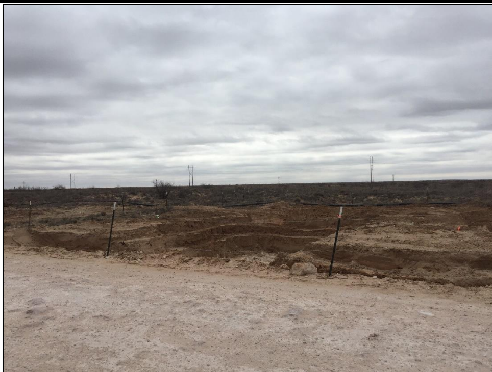
PHOTO 12: View of HA-4, HA-8, GP-4, Excavation, facing southeast. 02/19/2020 / TIME: 2:08PM / GPS: 32.6085 -103.4917
