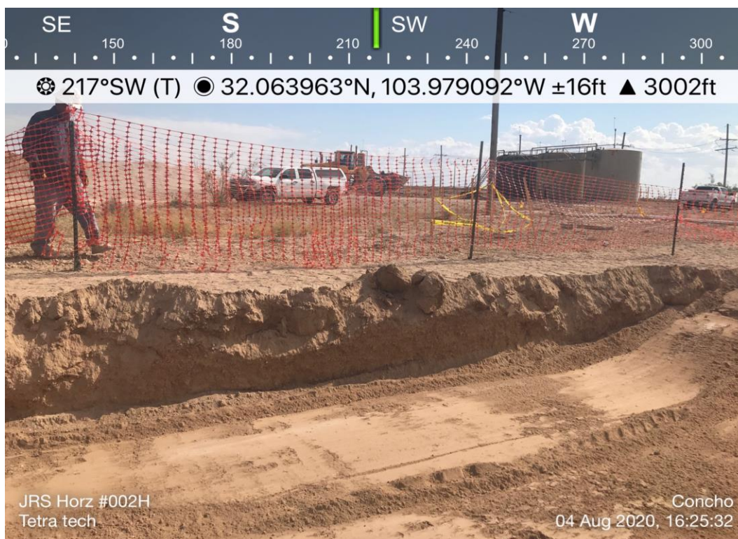
View Southwest – Remediated Area of AH-1
