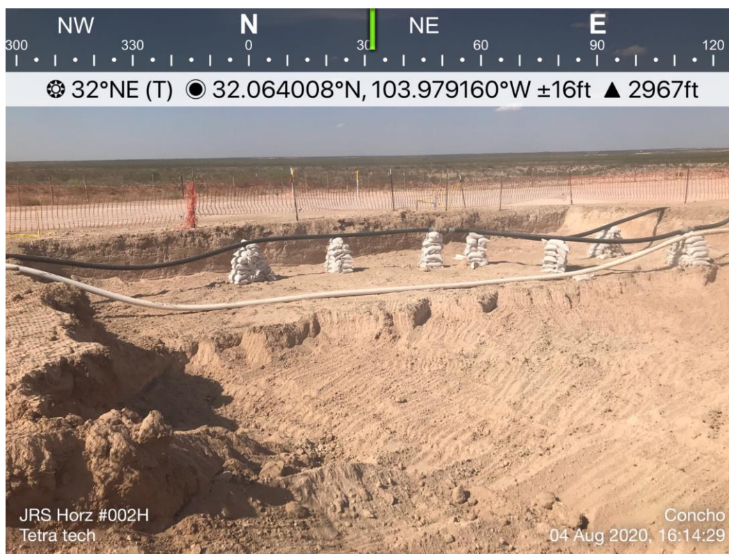
View Northeast – Remediated Area of AH-2 and AH-3
