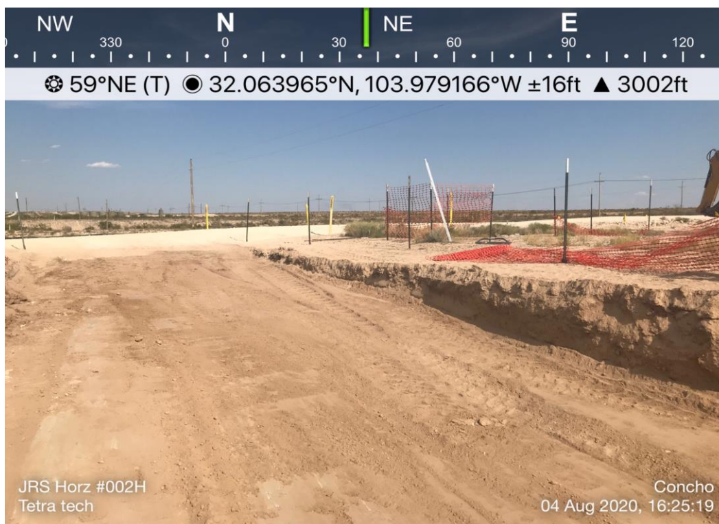
View Northeast – Remediated Area of AH-1
