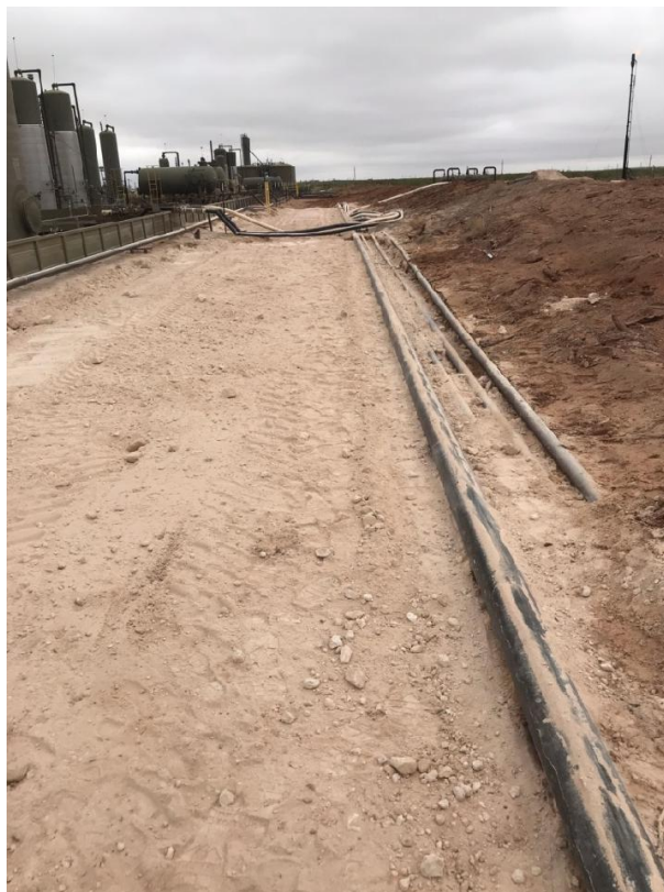
Photo of Backfilled area
