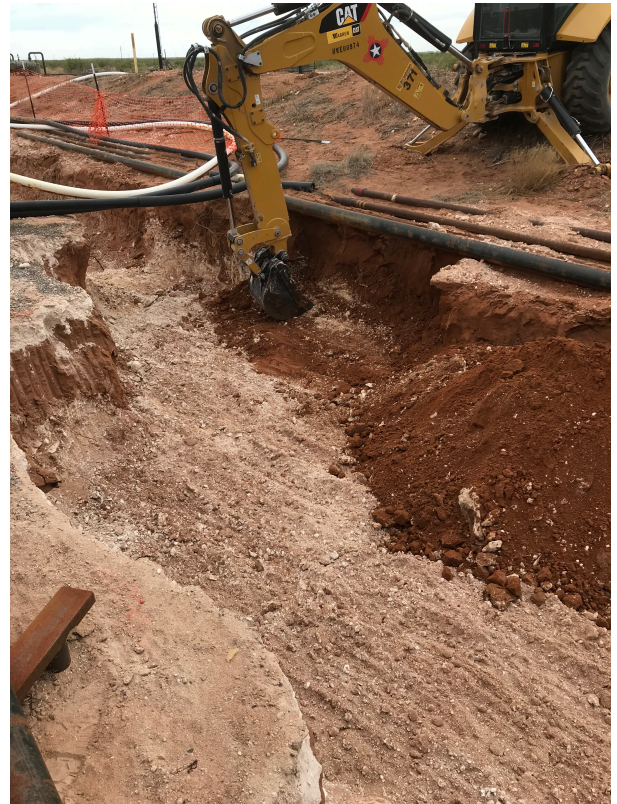
Photo of Excavation
