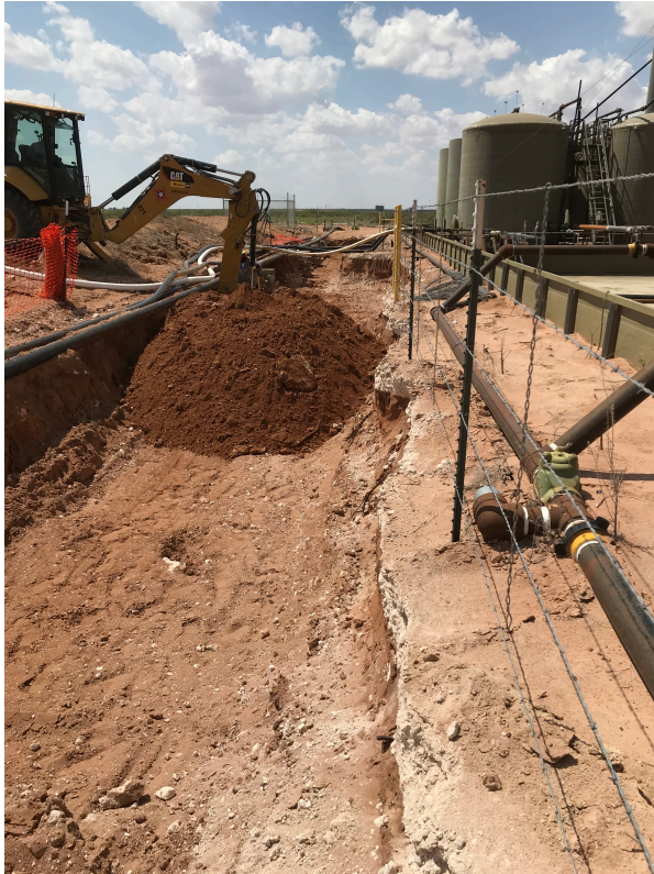
Photo of Excavation
