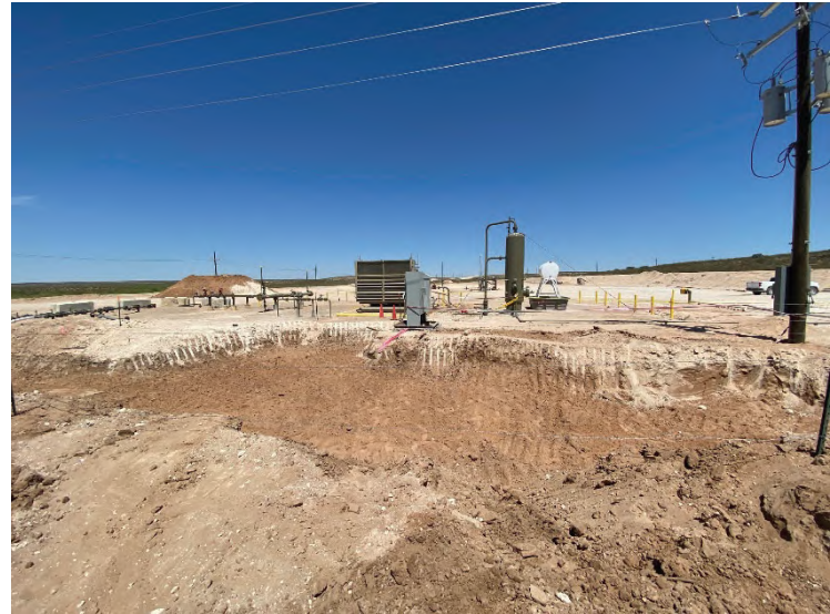
Photograph 4: Eastern view of excavation on pad.
