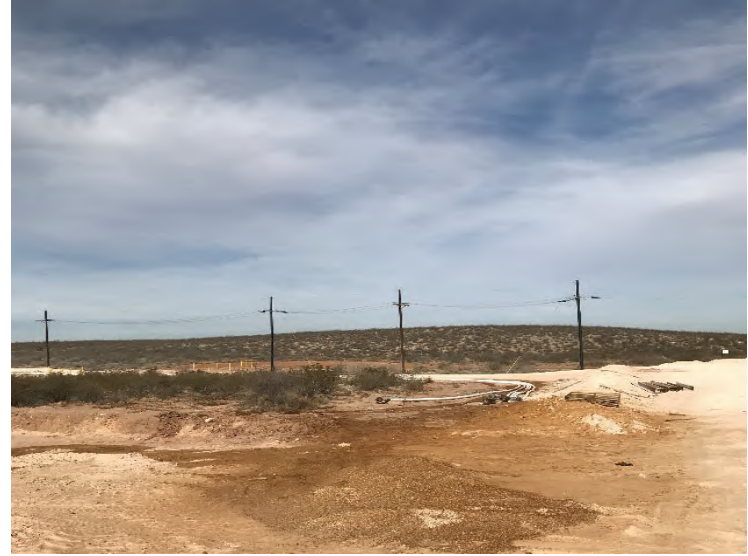
Photograph 2: North western view of stained area.
