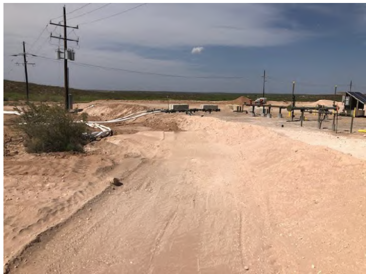
Photograph 7: Northern view of backfilled excavation.
