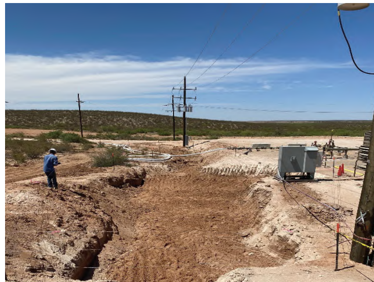
Photograph 6: Northern view of excavation.
