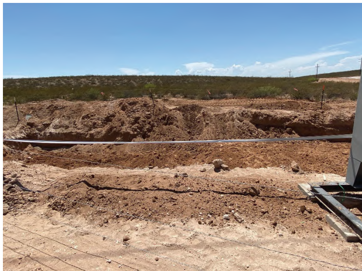
Photograph 5: Western view of excavation on pad.
