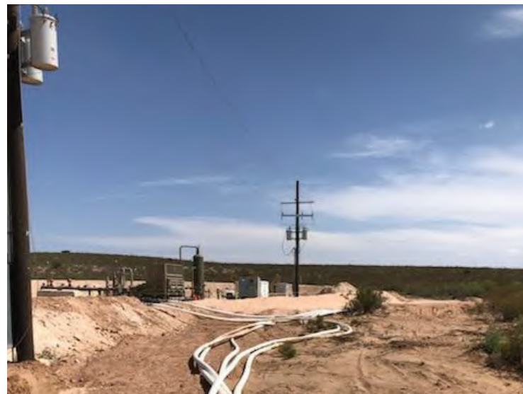
Photograph 8: Southern view of backfilled excavation.
