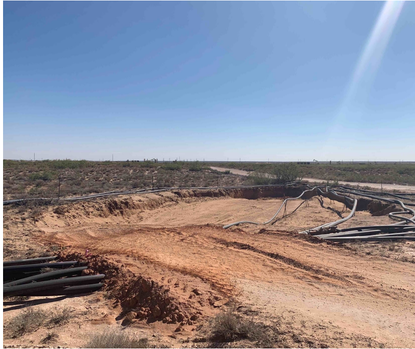
Photo of Excavation
