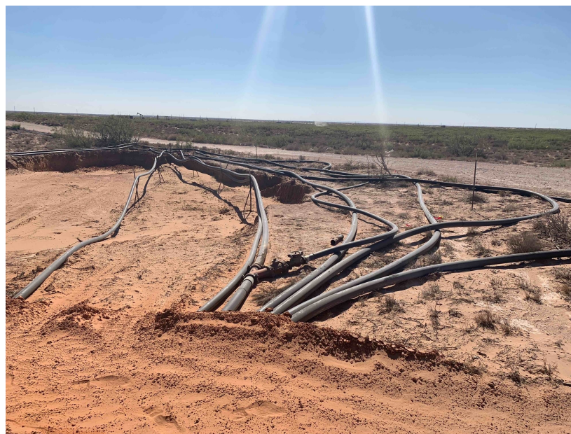
Photo of Excavation
