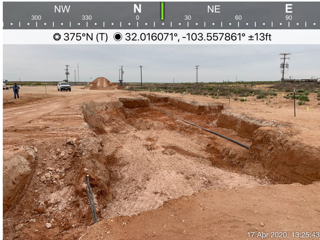
View of Remediation – View North
