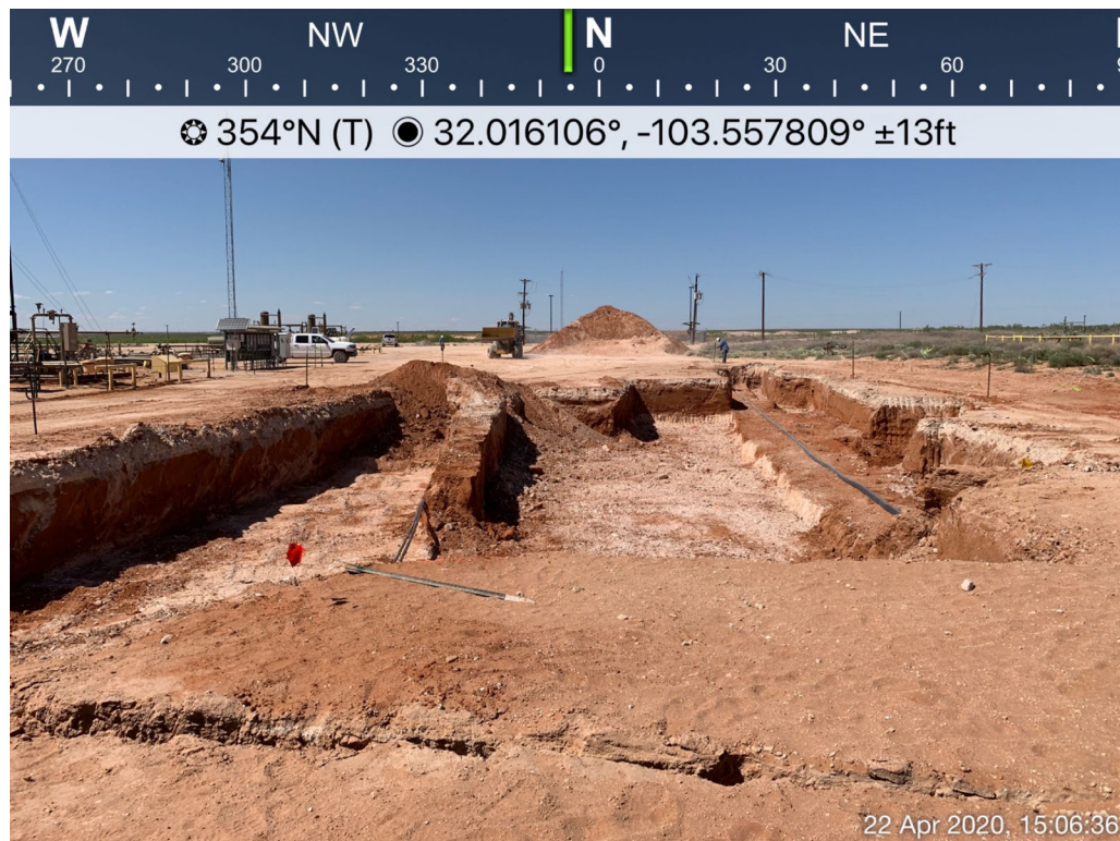
View of Remediation – View North
