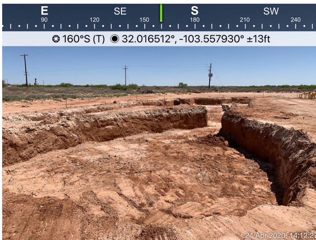
View of Remediation – View South/Southeast
