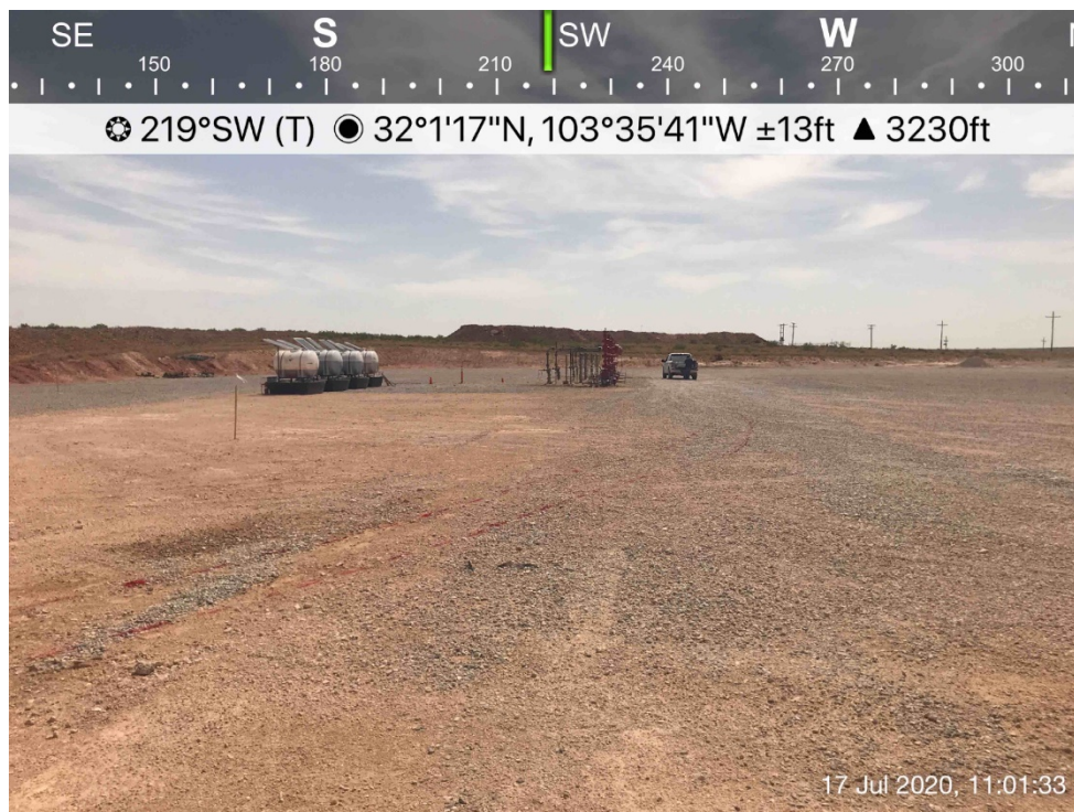
Impacted area viewing southwest, July 17, 2020
