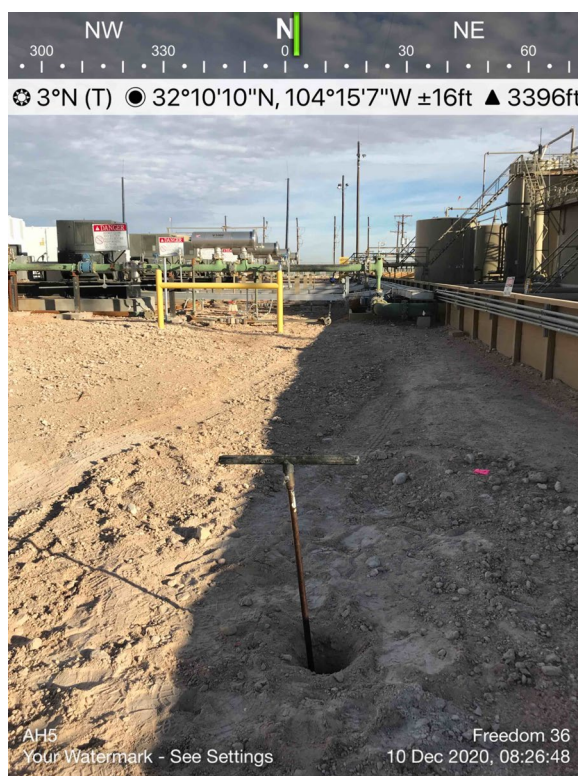
View of Release Area – View North
