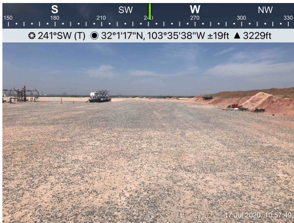
Impacted area viewing southwest, July 17, 2020
