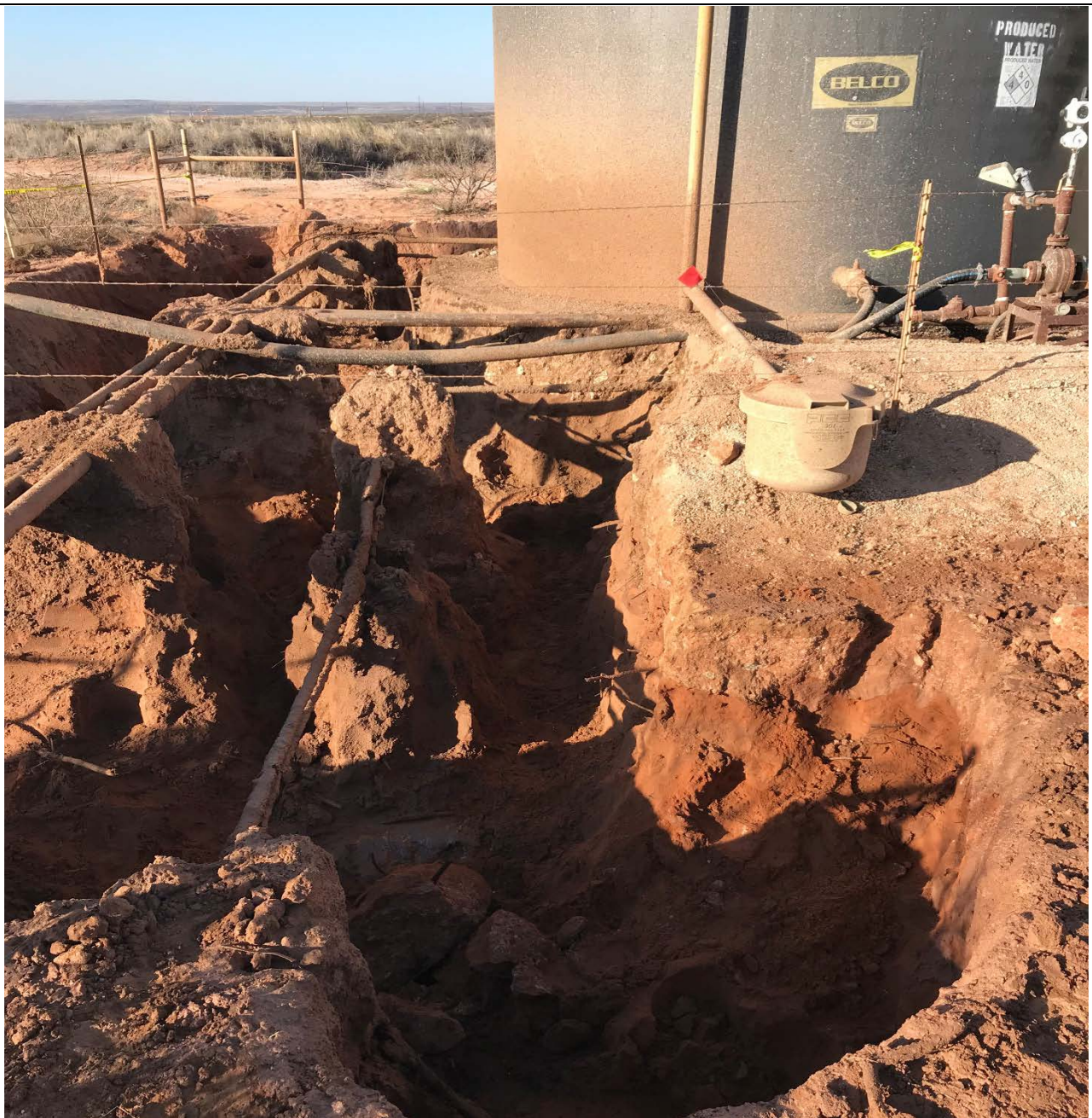
View facing north of initial excavation activities.
