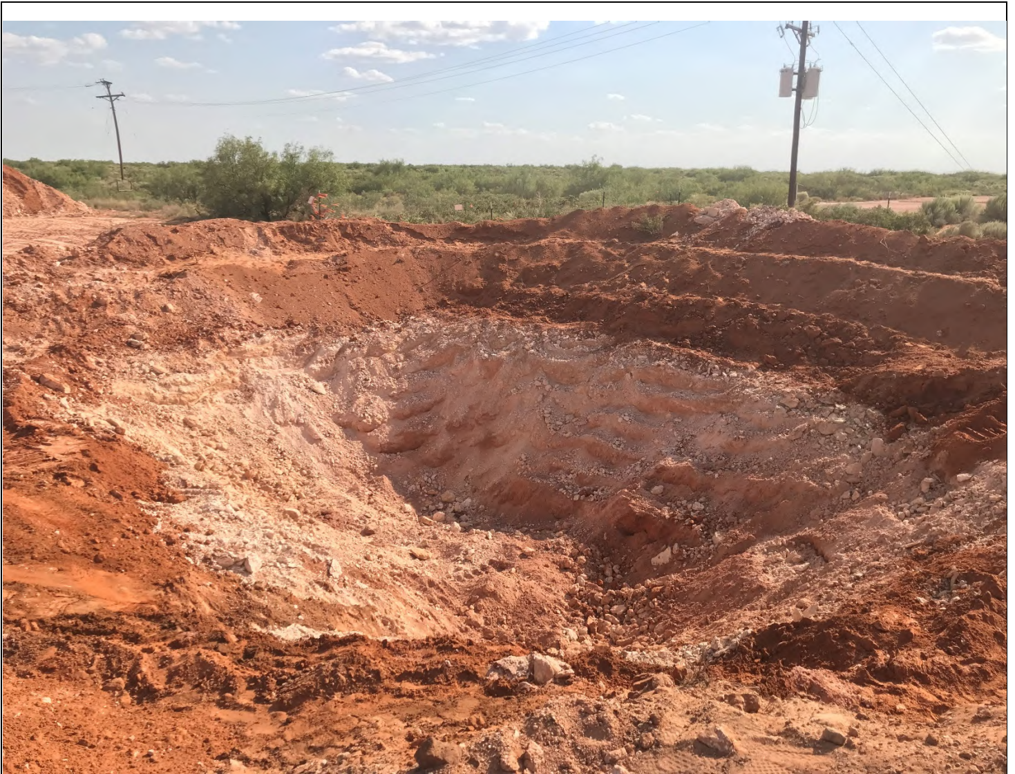
View facing southwest of the open excavation.
