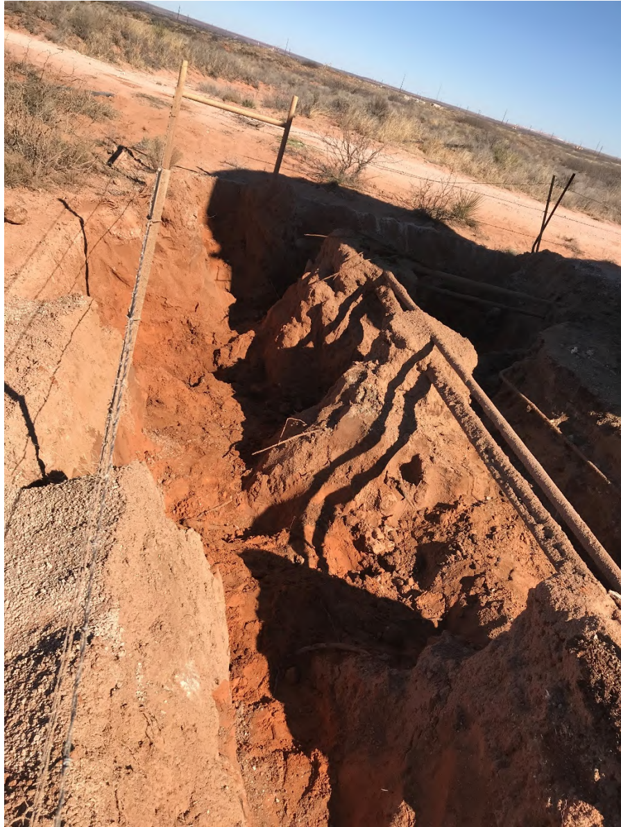
View facing west of initial excavation activities.
