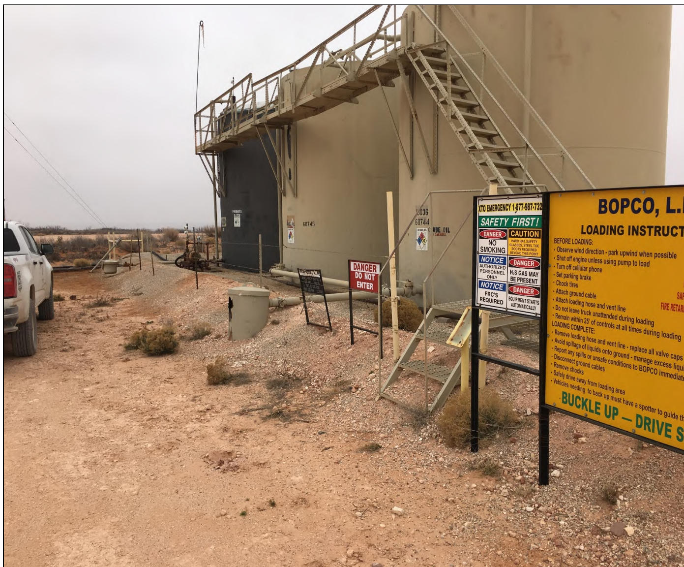
View facing northwest of earthen berm around tank battery.
