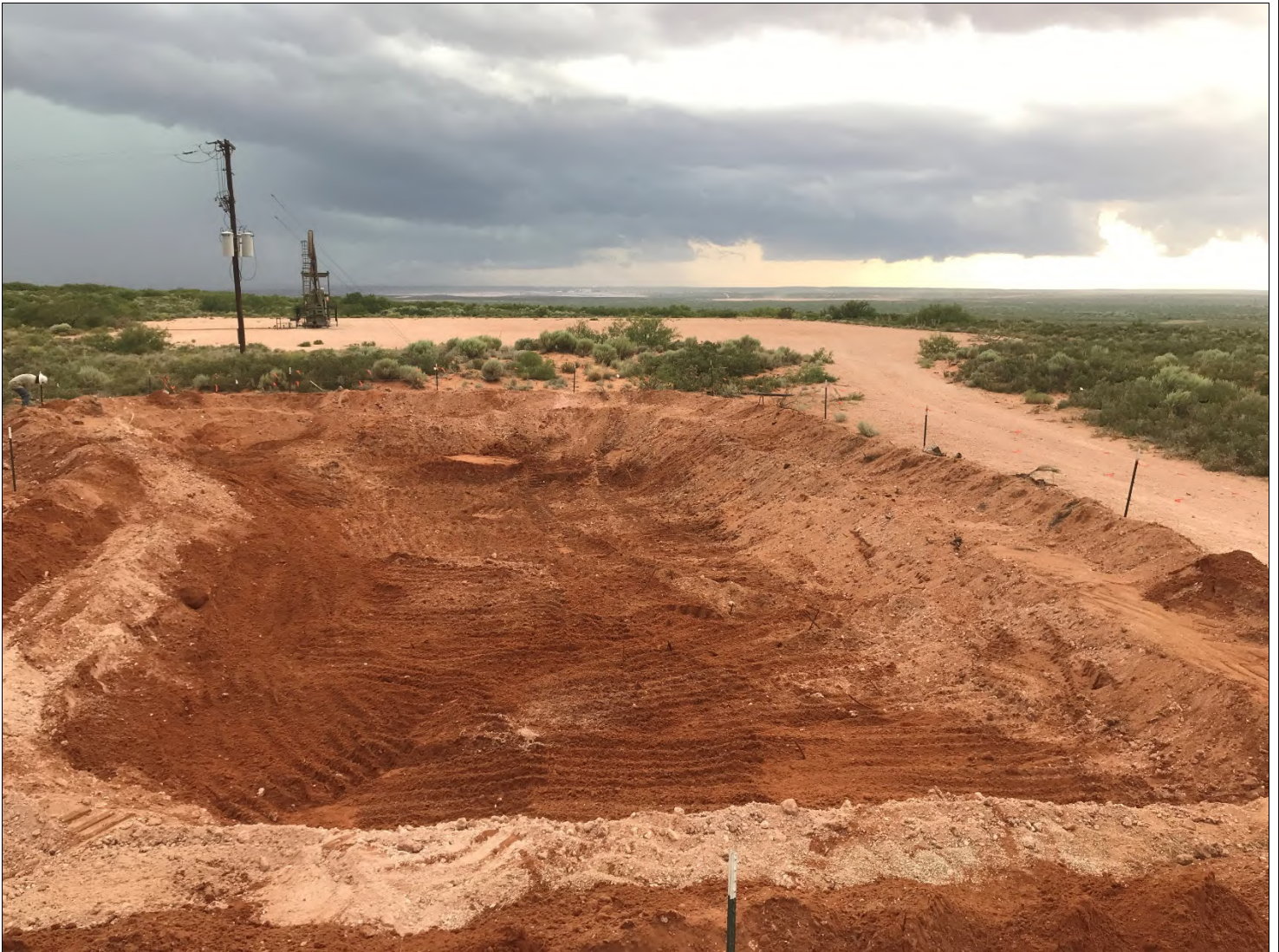
View facing west post tank battery removal.
