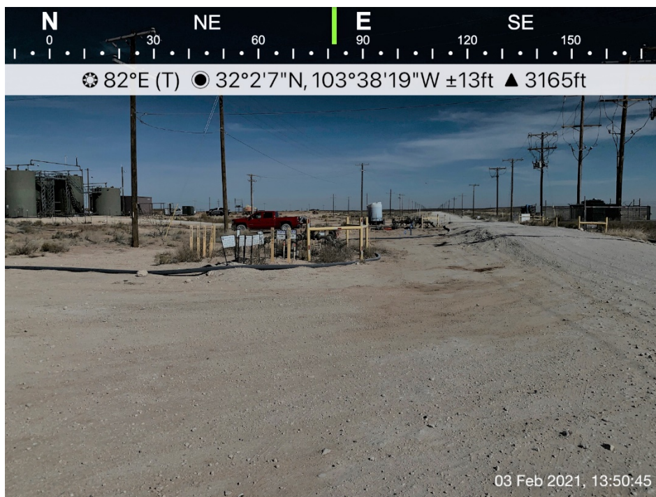
Impacted area viewing East, February 3, 2021
