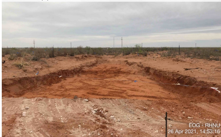
View of Remediation Activities – View West
