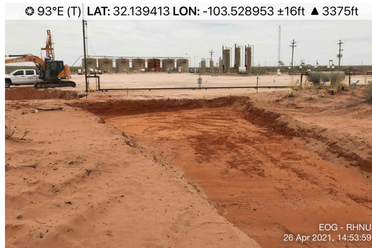
View of Remediation Activities – View East
