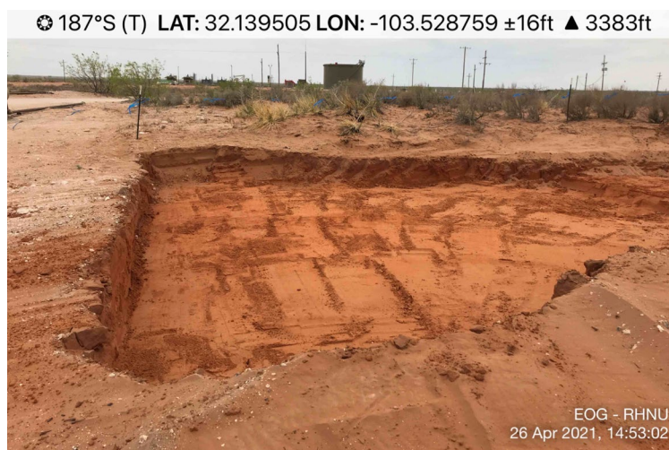
View of Remediation Activities – View South
