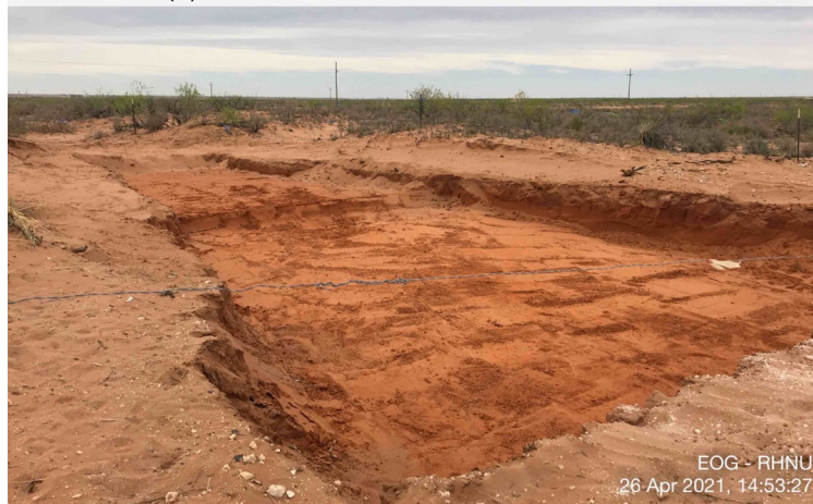
View of Remediation Activities– View Northwest
