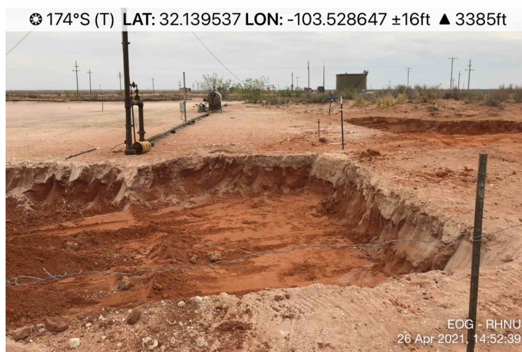
View of Remediation Activities – View South
