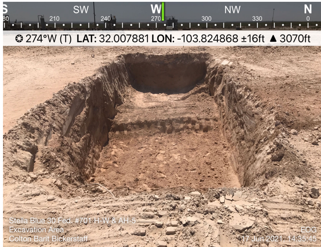
View of Remediation Activities – View West
