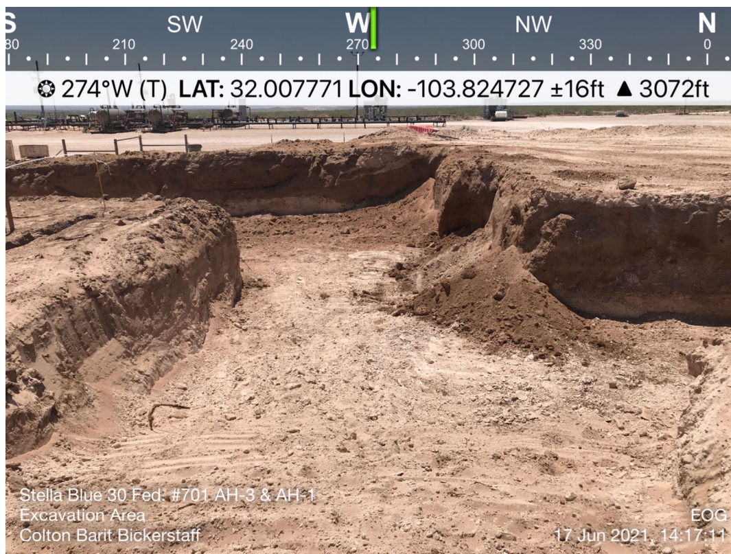
View of Remediation Activities – View West
