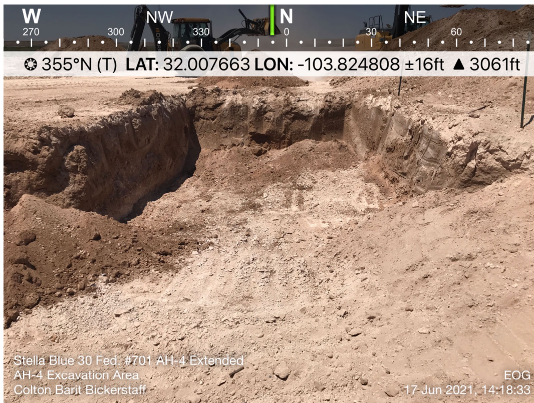
View of Remediation Activities – View Northwest/North
