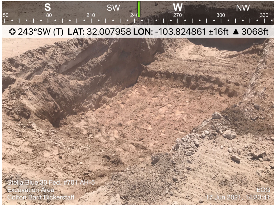
View of Remediation Activities – View Southwest
