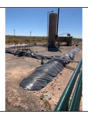
The liner was visually inspected and no rips, tears, holes, or damage in the liner was observed. The liner was determined to be in good condition.
