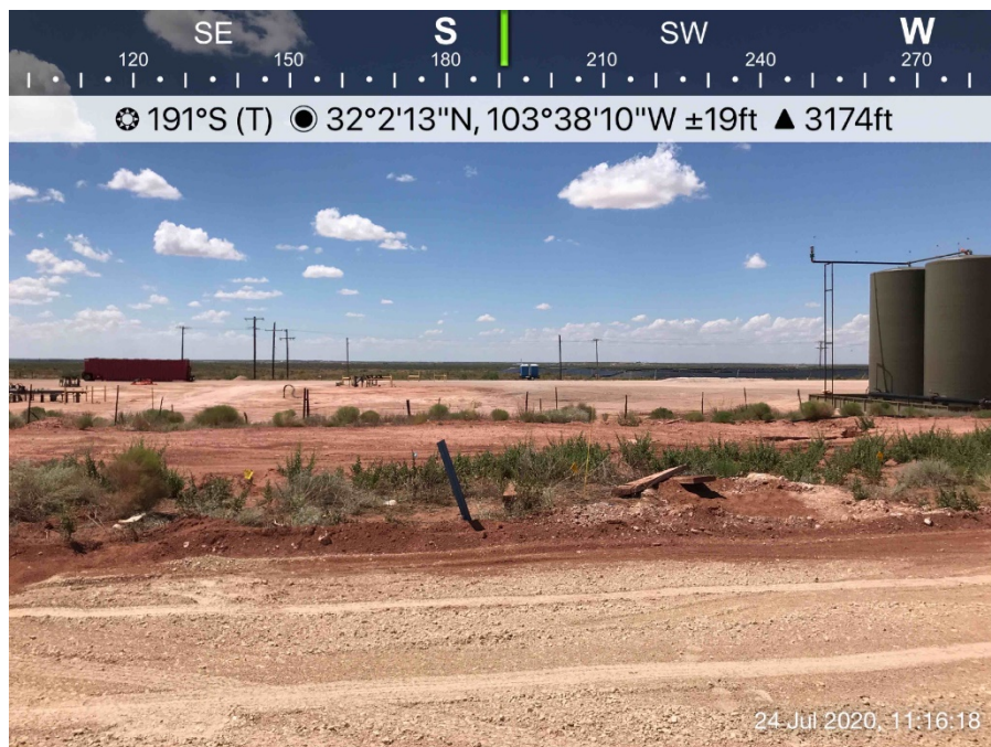
View to the south of the spill area from the frac ponds prior to remediation.
