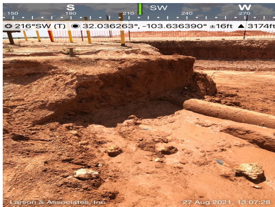
View to the southwest of the pipeline and southern sidewall, and includes the southern 4.1' section of the excavation.
