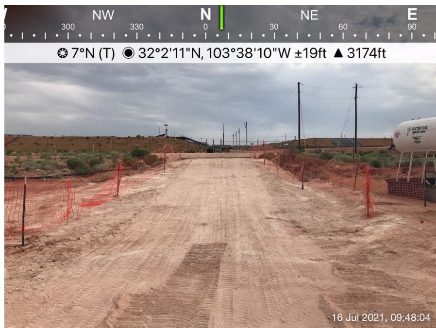
View of the ramp leading to the frac ponds, which was removed and replaced with clean soil.
