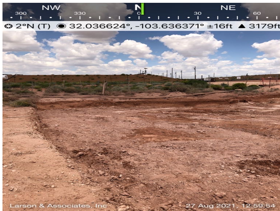
View to the north of the northern 2' excavated area.
