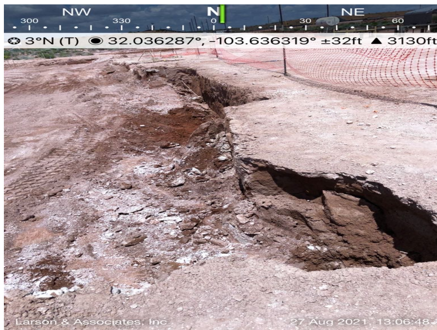
View to the north of the eastern sidewall (4.1') of the most southern portion of the excavation.
