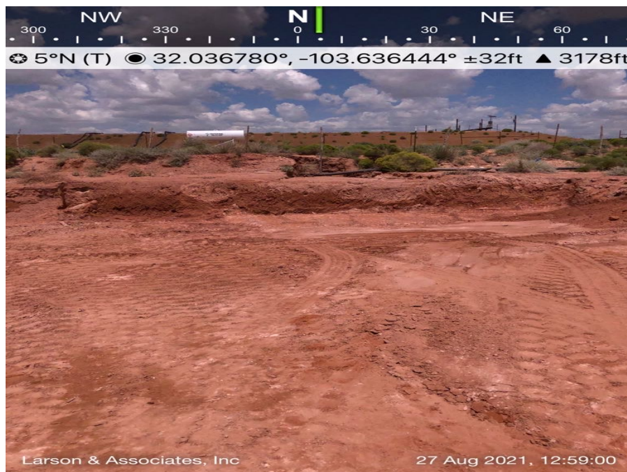
View to the north of the northern 4.1' excavated area.
