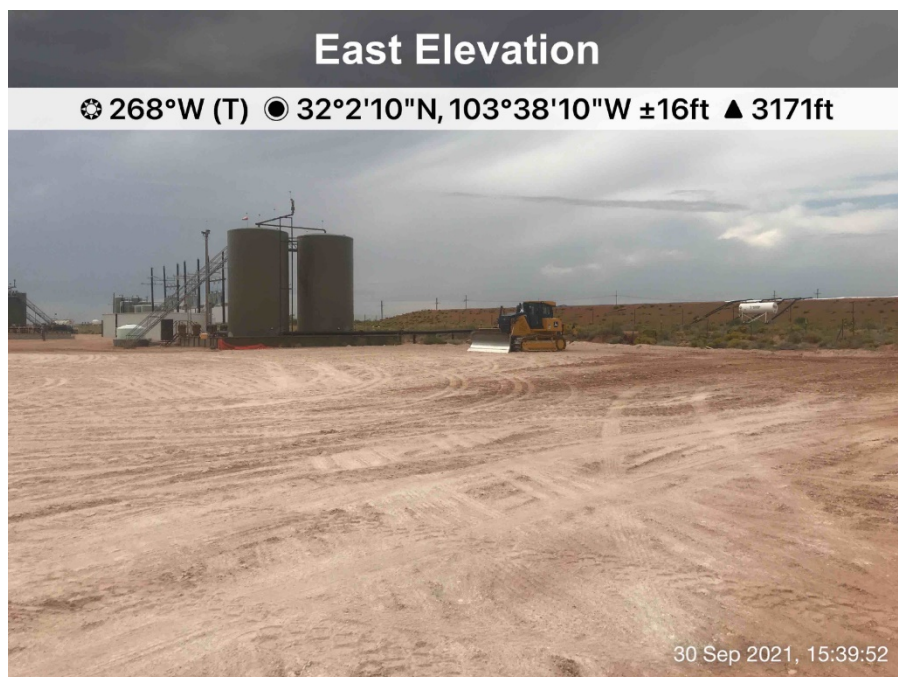
View to the northwest of the site after being backfilled.
