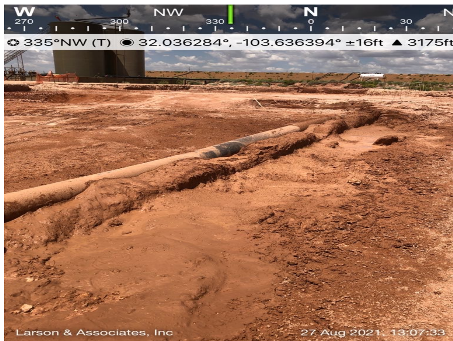
View to the north - northwest of the pipeline (within the southern 4.1' area), which is in the center of the excavation.
