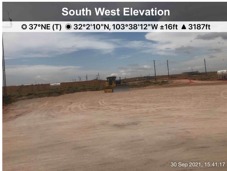
View to the north of the site after being backfilled.
