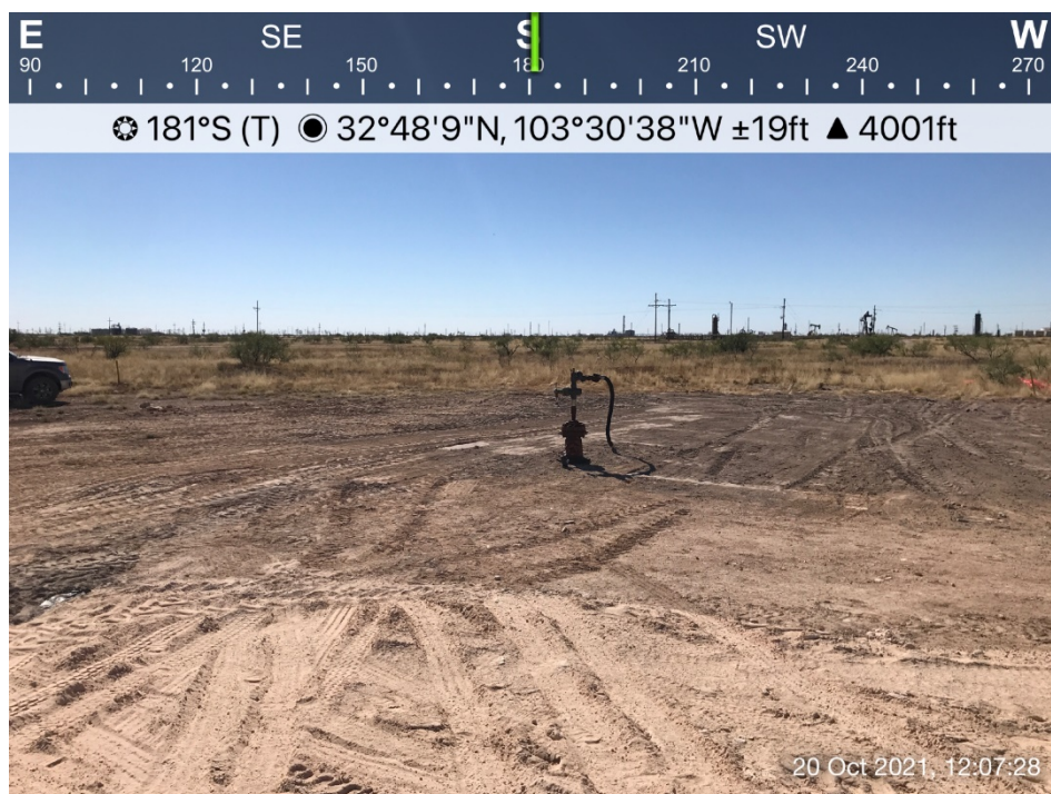
Backfilled Excavation Area Encompassing S-4
