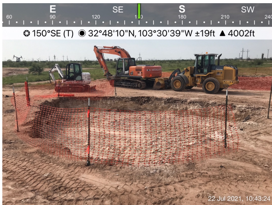
Excavated Soil Encompassing S-6 and S-9 to a depth of 4.1 Feet bgs
