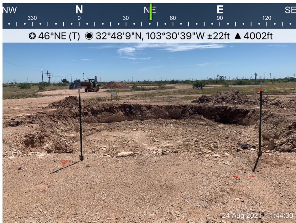
Additional 1-foot Excavated from the Sidewall Encompassing C-18
