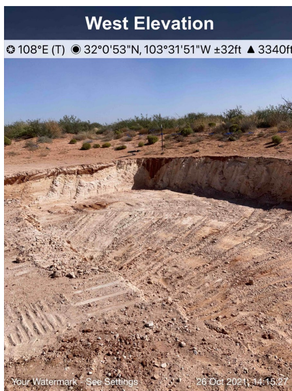
View of Remediation Activities – View East
