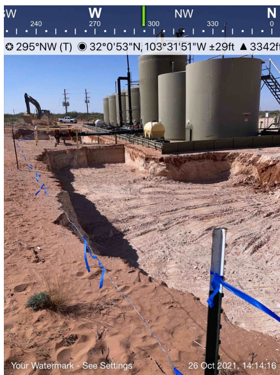
View of Remediation Activities – View Northwest
