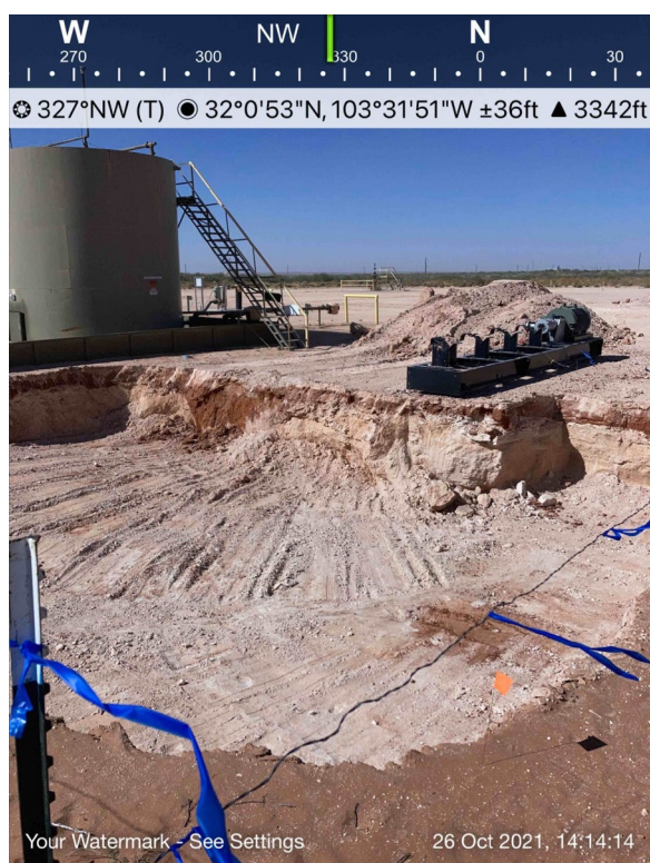
View of Remediation Activities – View Northwest
