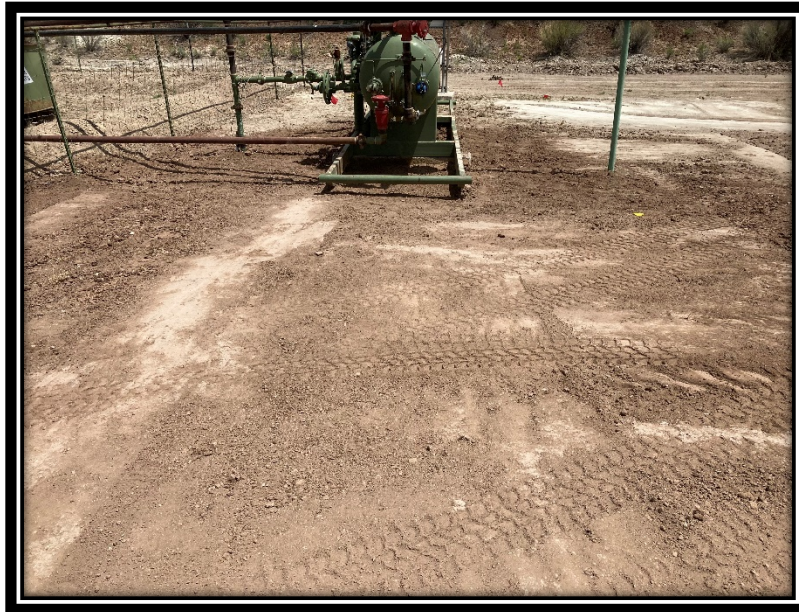
Picture 3: Backfilled Area (View 1)
