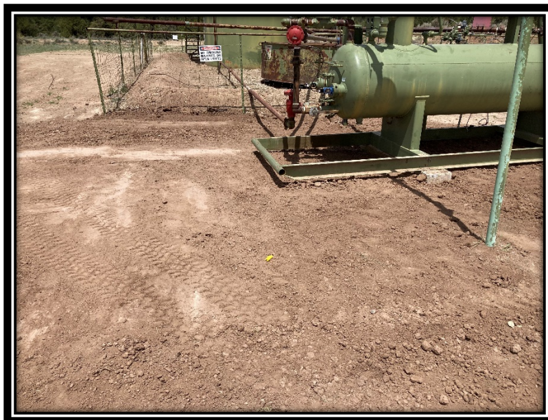
Picture 4: Backfilled Area (View 2)
