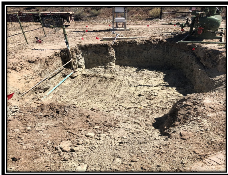
Picture 2: Excavation (View 2)
