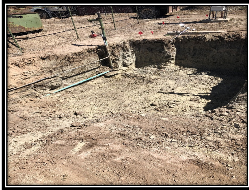
Picture 1: Excavation (View 1)
