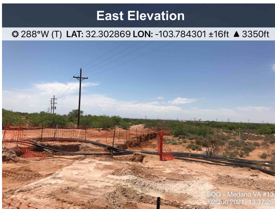
View of Remediation Activities – View West
