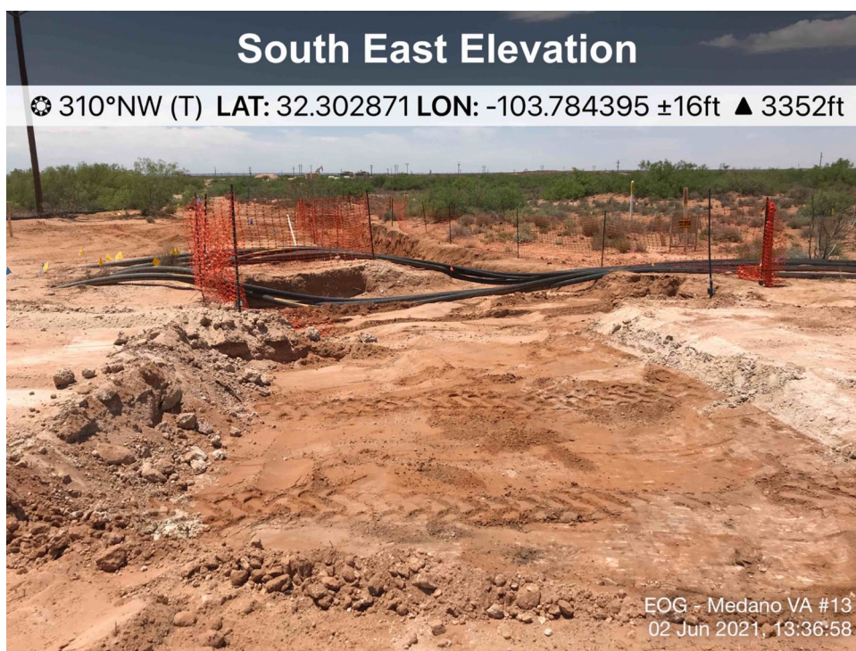
View of Remediation Activities – View Northwest
