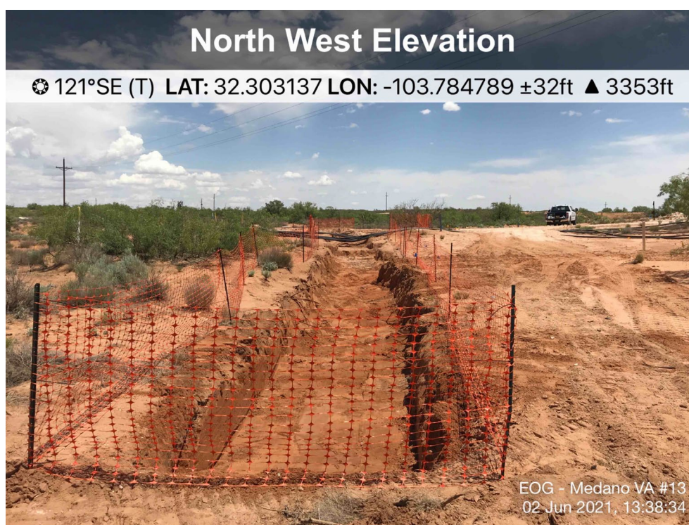
View of Remediation Activities – View Southeast
