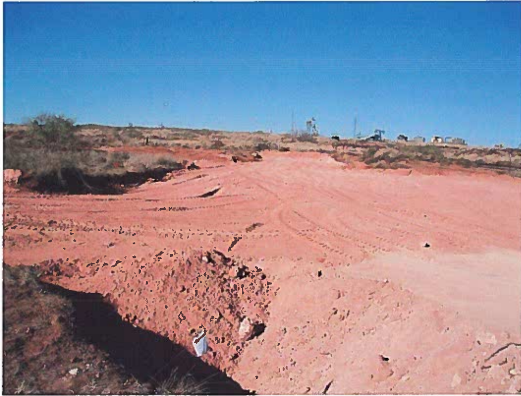
View West – Backfilled area of SB-1 and SB-5
