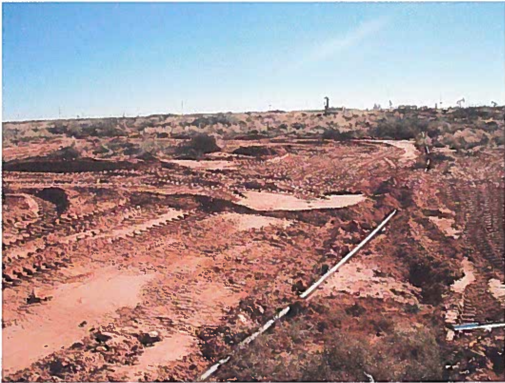
View South– Backfilled area of SB-9 and SB-4
