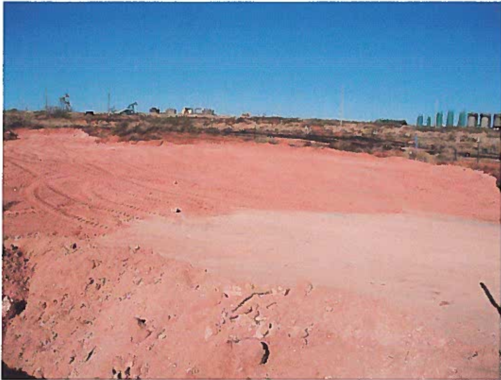
View North – Backfill area of SB-1 and SB-5
