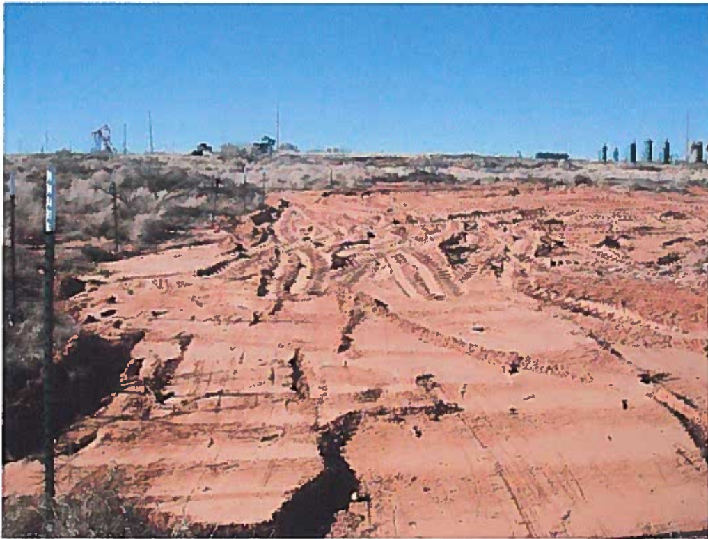
View West – Backfill area of AH-5 and SB-5
