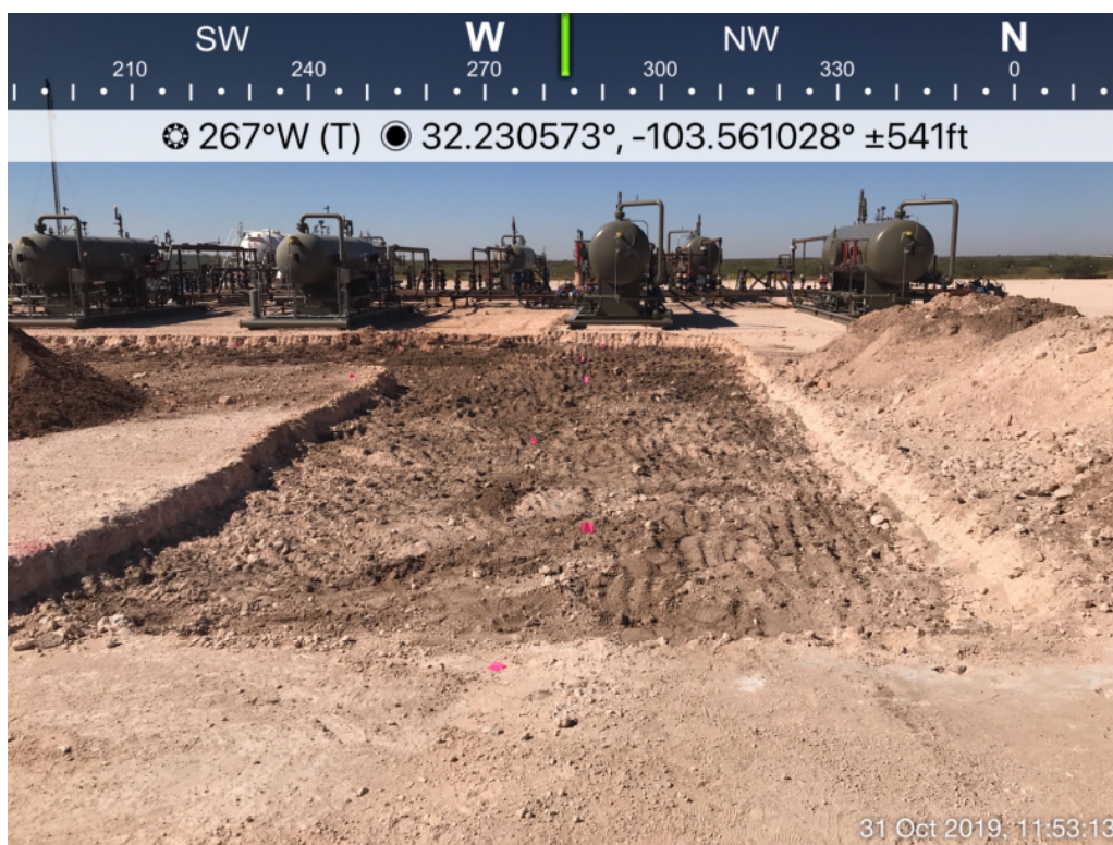
View West – Excavated Area of AH-6
