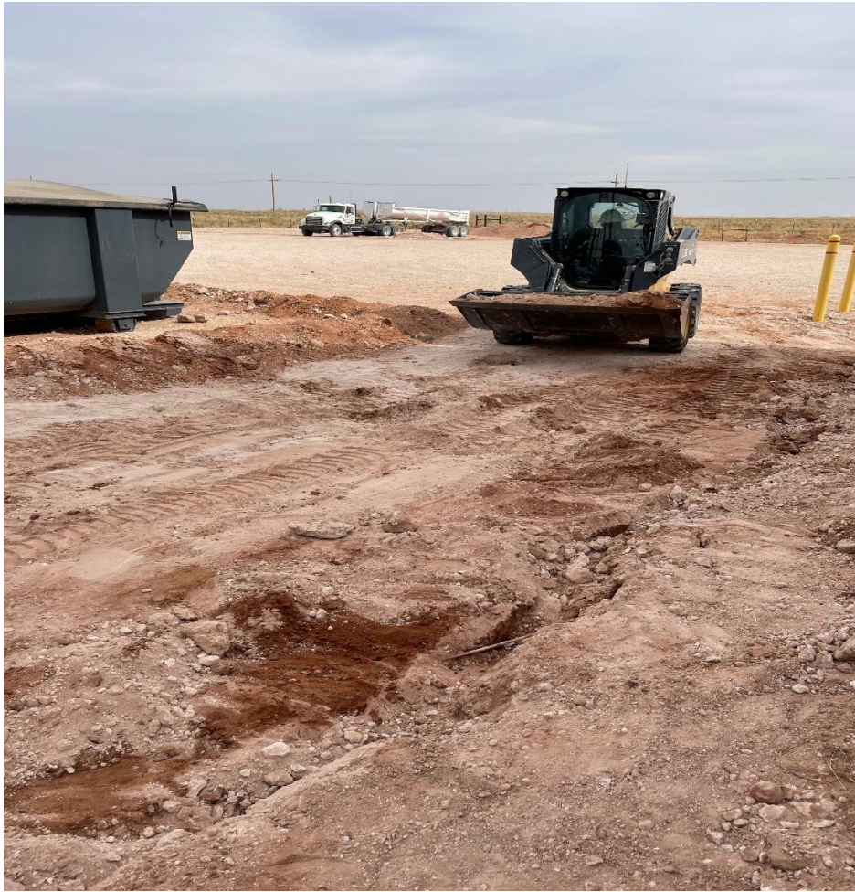
Figure 10: Image of excavation done on quadrants 2-4
