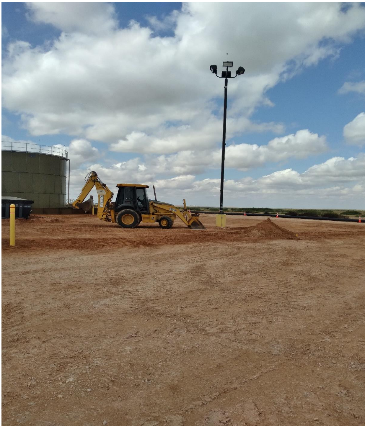
Figure 6: Removal of Top Layer of Contaminated Soil Using Backhoe
