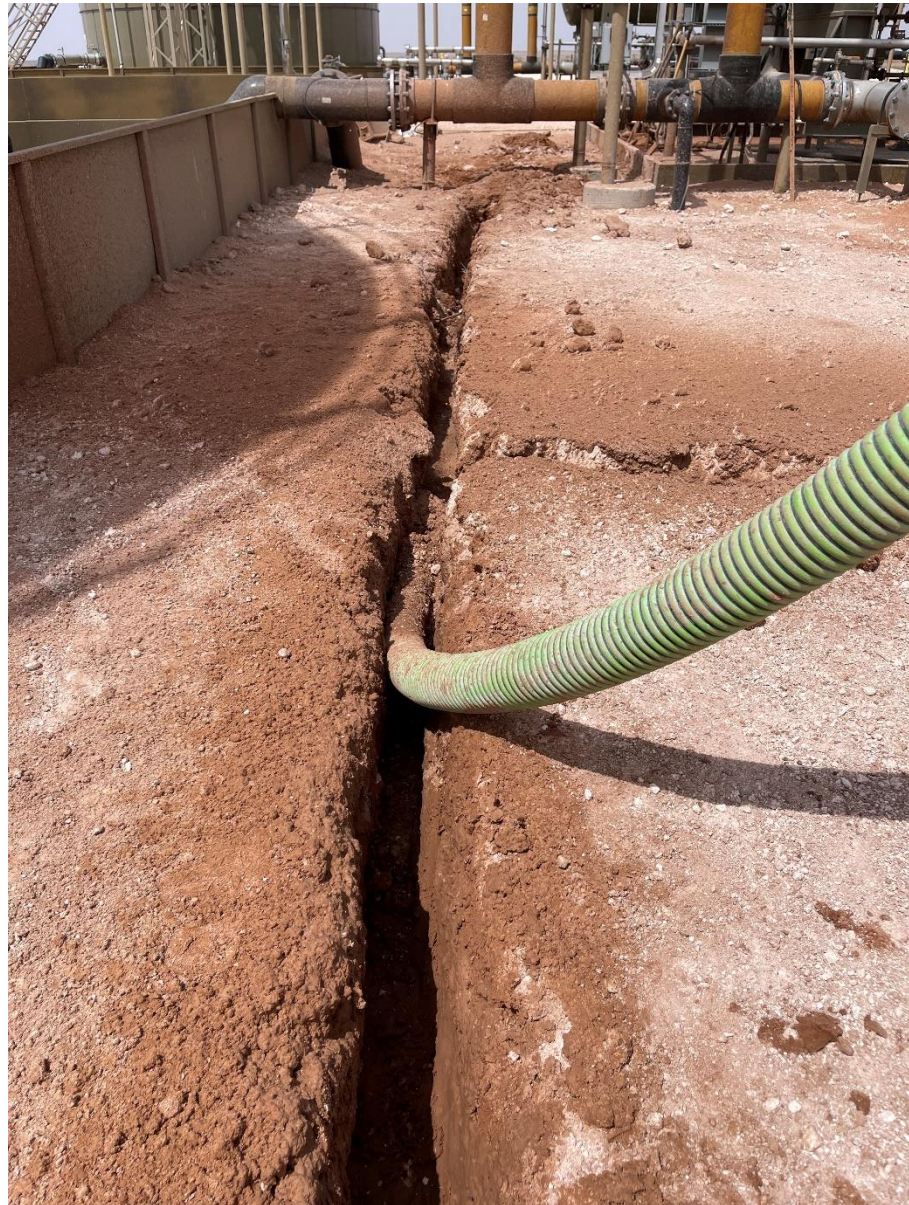
Figure 9: Image of daylighting done on quadrants 2-4 for additional excavation required
