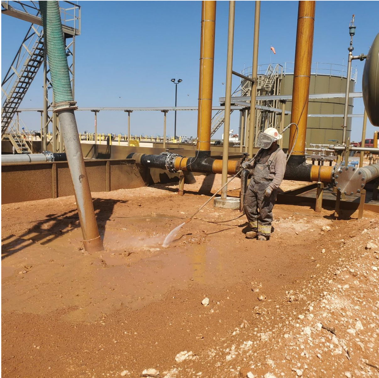
Figure 5: Removal of Top Layer of Contaminated Soil Using Hydro-Vac
