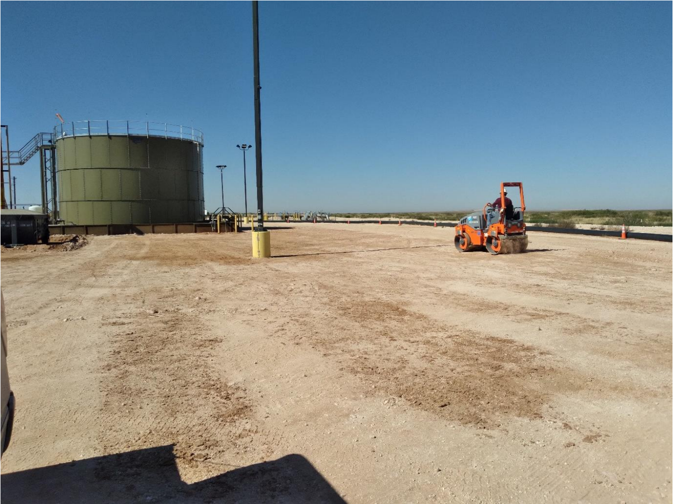
Figure 12: Rolling of Clean Soil Brought in for Replacement
