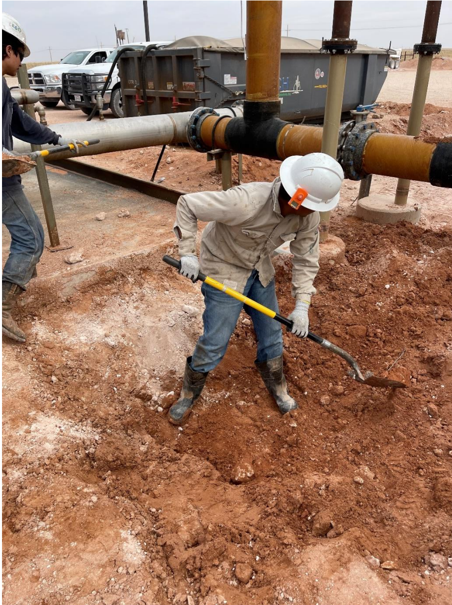
Figure 11: Supplemental image of Excavation done on quadrants 2-4
