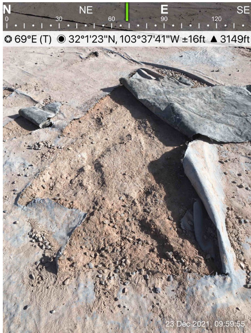
View of torn liner, December 23, 2021
