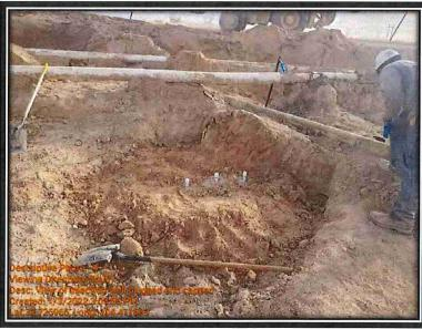
Picture 4: 01/03/2022 Plugged and capped Vent Wells.
