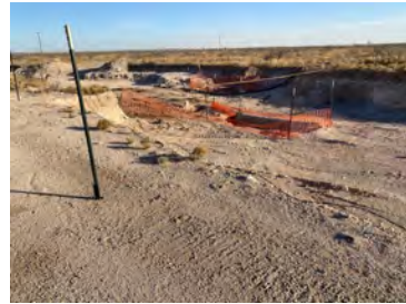
View of E of W excavation at proposed liner area (1/18/22).
