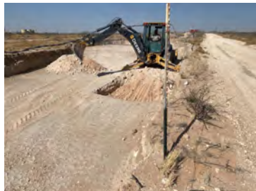
Excavation at C-137 (4/18/22).
