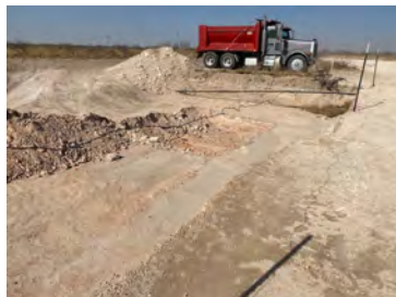
View of excavation at C-64 (4/18/22).
