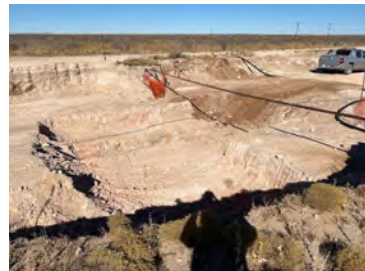
View to N of proposed liner area at W excavation (2/7/22).
