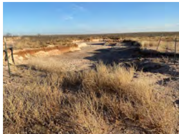
View to S of E excavation (1/18/22).
