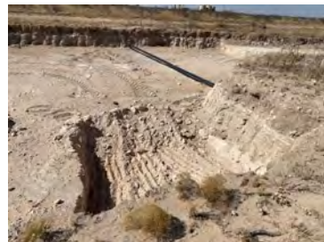
Excavation at C-116 (4/18/22).
