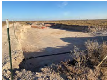
View to E of W excavation (1/18/22).
