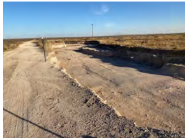
View to E of W excavation (E of proposed liner area). 1/18/22
