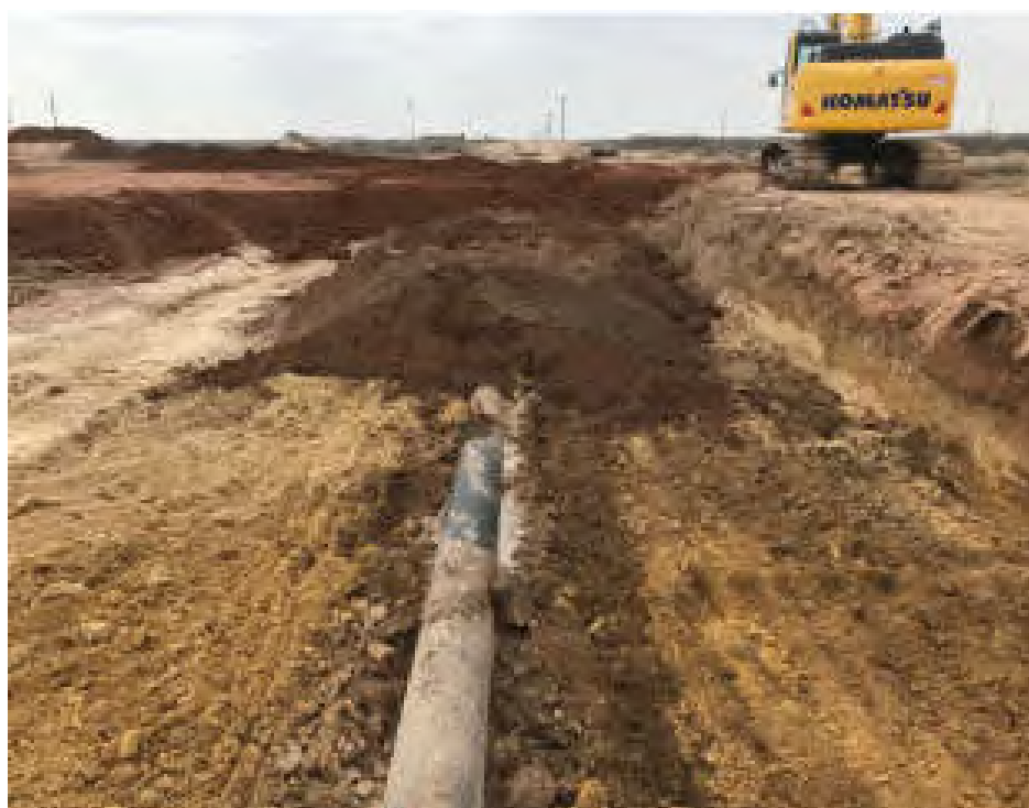
Photo 10: View during the placement of backfill above the buried pipeline.
