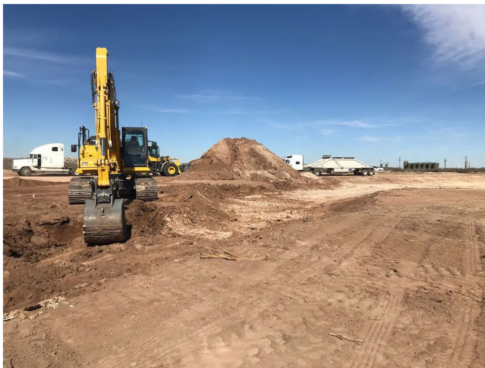
Photo 3: View of excavation of impacted soil.
