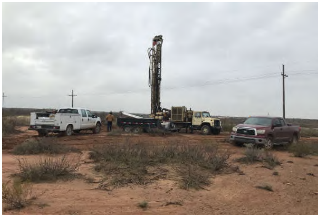
Photo 7: View of the drilling of the temporary water well to 62 feet (dry).
