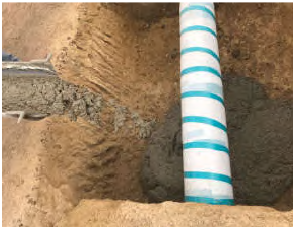
Photo 9: View of the placement of flowable fill to support the pipeline prior to backfilling.
