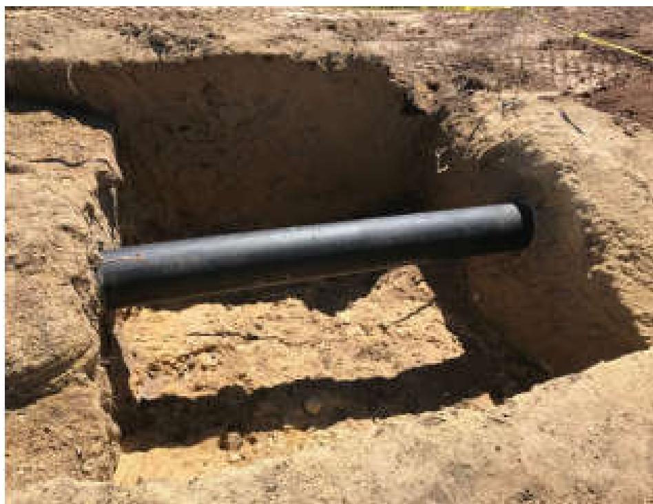
Photo 8: View of a portion of the excavated area around the buried pipeline.
