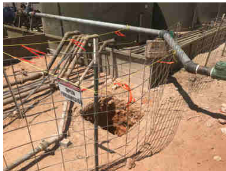
Photograph 8: View of open excavation (2RP-3985).
