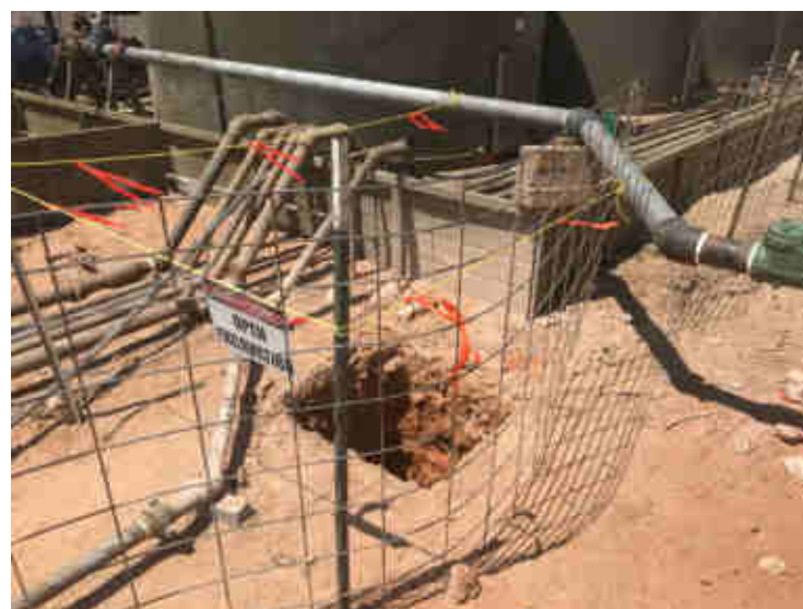
Photograph 8: View of open excavation (2RP-3985).
