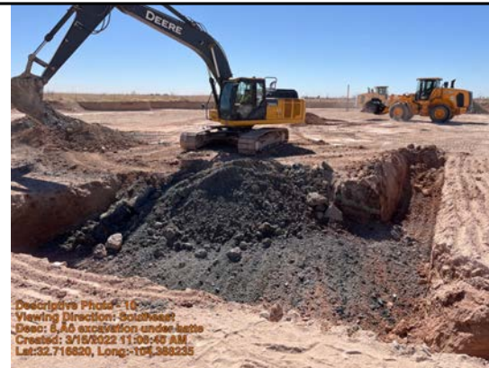
8' excavation under sample points 38 and 41
