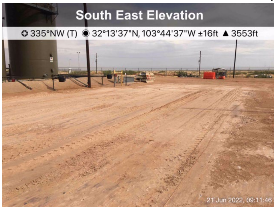
Backfilled excavation (nAPP2106659781) viewing northwest
