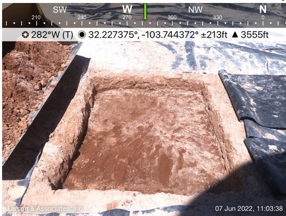
Excavated soil (nAPP2205652777) viewing West
