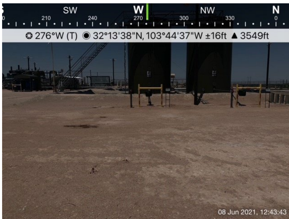
Spill Area (nAPP2106659781) viewing West
