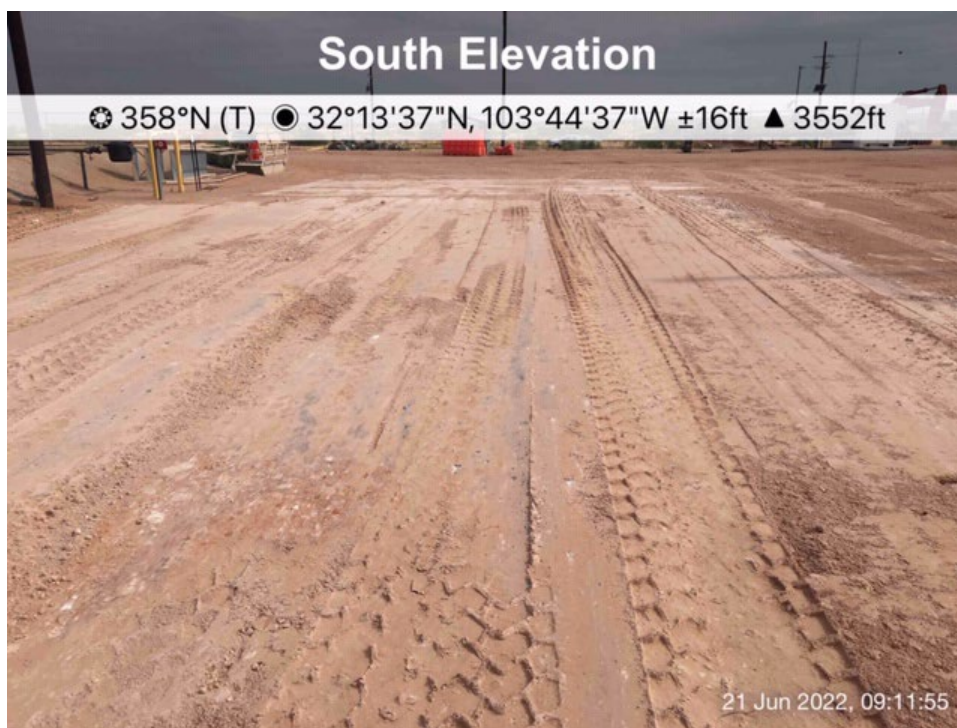
Backfilled excavation (nAPP2106659781) viewing north
