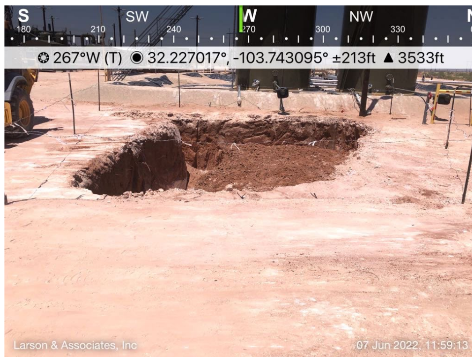
Excavated soil (nAPP2106659781) viewing West
