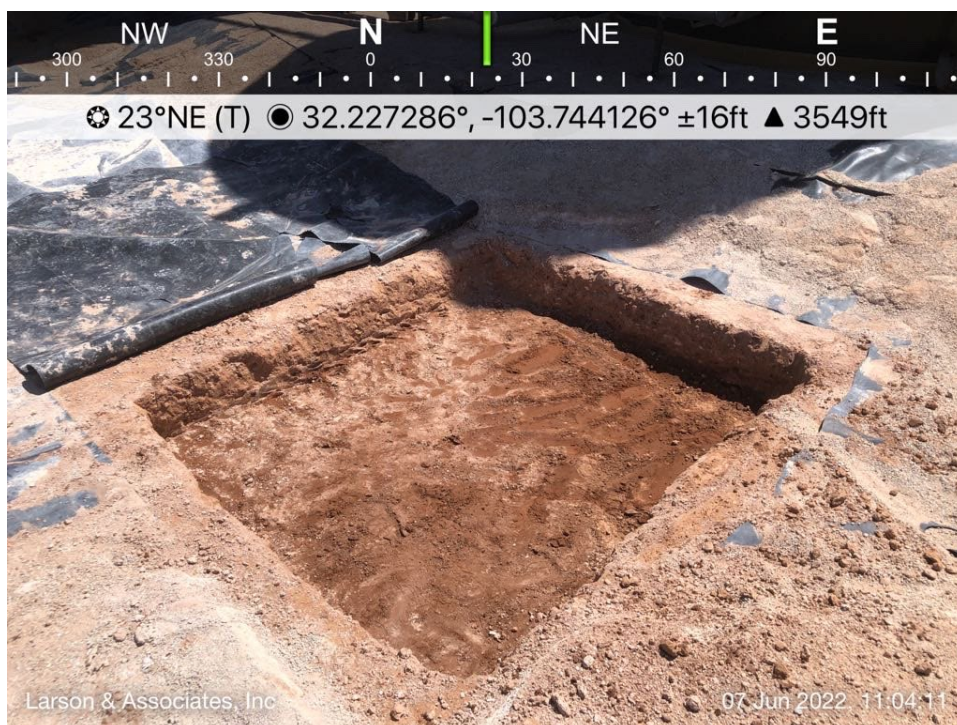
Excavated soil (nAPP2205652777) viewing Northeast
