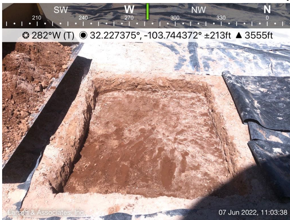
Excavated soil (nAPP2205652777) viewing West
