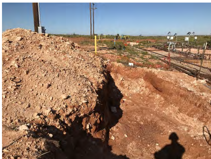
Photograph 11: View of open excavation (2RP-4398), facing west.
