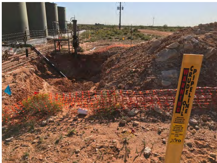
Photograph 9: View of open excavation (2RP-4398), facing east.
