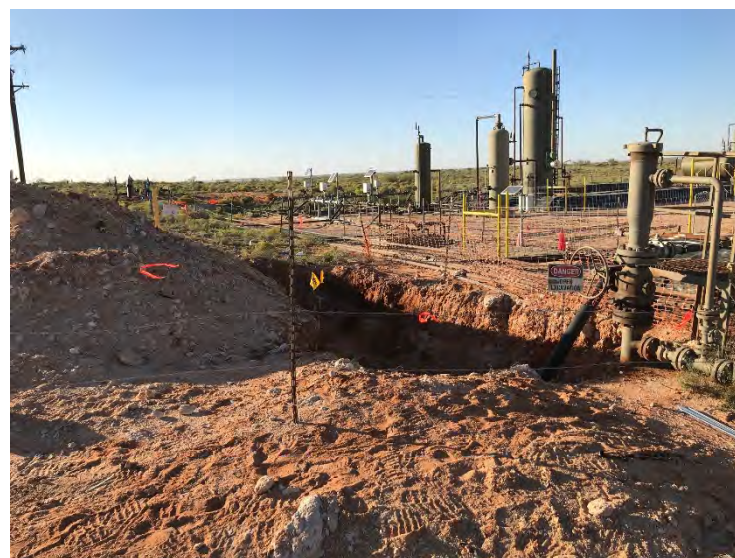
Photograph 12: View of open excavation (2RP-4398), facing northwest.
