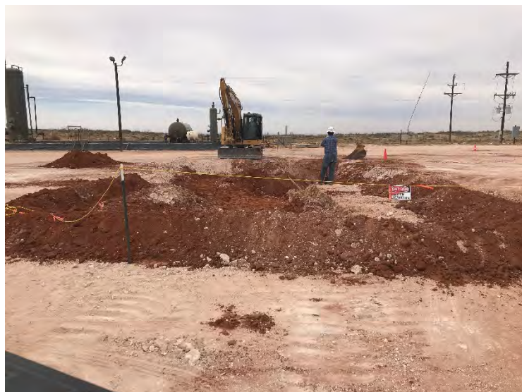
Photograph 3: View of excavation (2RP-2526), facing west.
