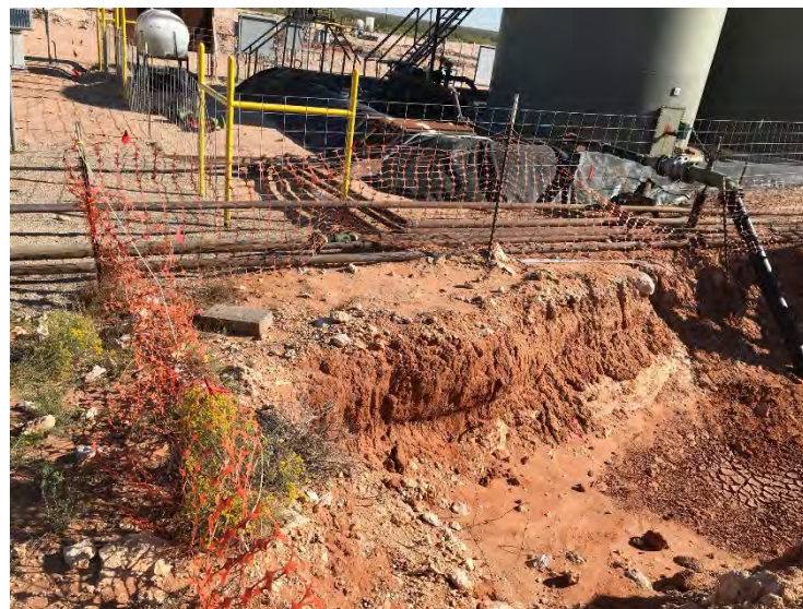
Photograph 10: View of open excavation (2RP-4398), facing north.
