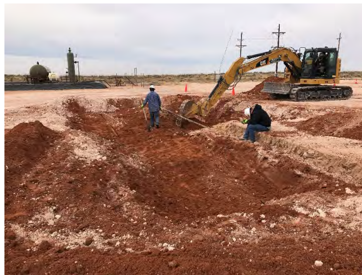
Photograph 2: View of excavation (2RP-2526), facing west.
