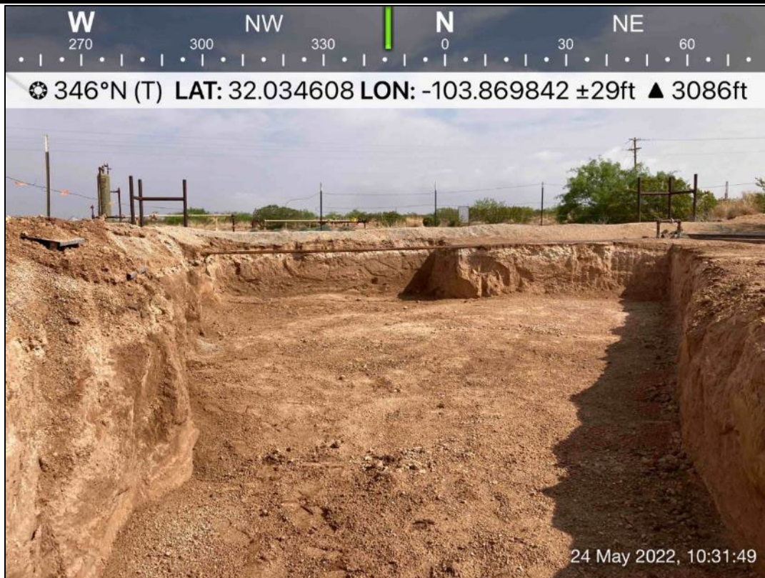
PHOTO 6: View of the excavated area facing north. 5/24/2022
