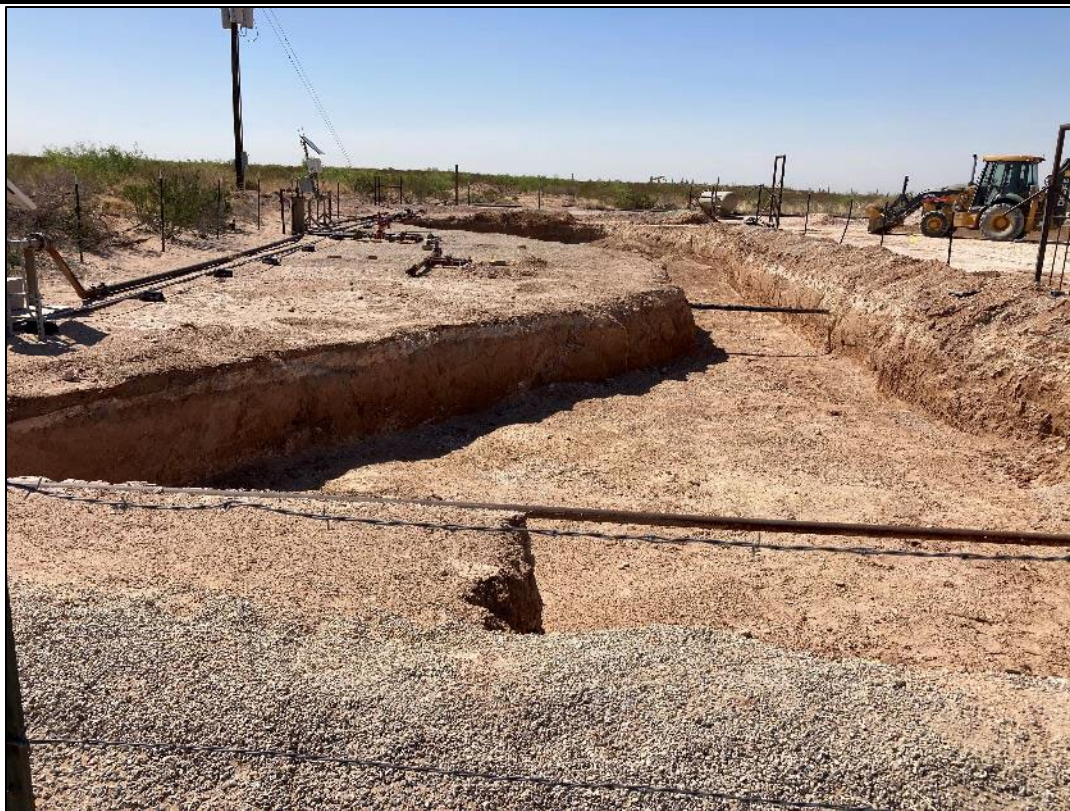
PHOTO 11: View of the excavated area facing south. 5/26/2022
