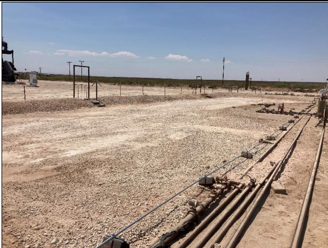
PHOTO 17: View of the remediated area facing northwest. 5/27/2022
