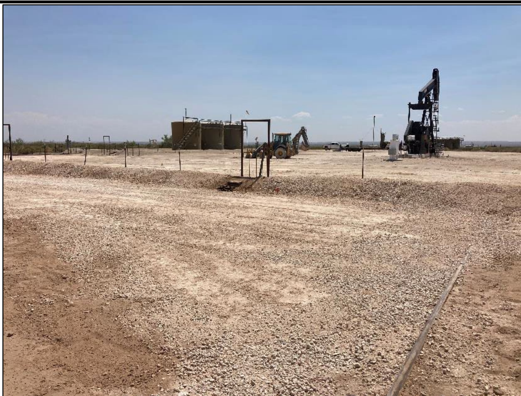
PHOTO 20: View of the remediated area facing southwest. 5/27/2022
