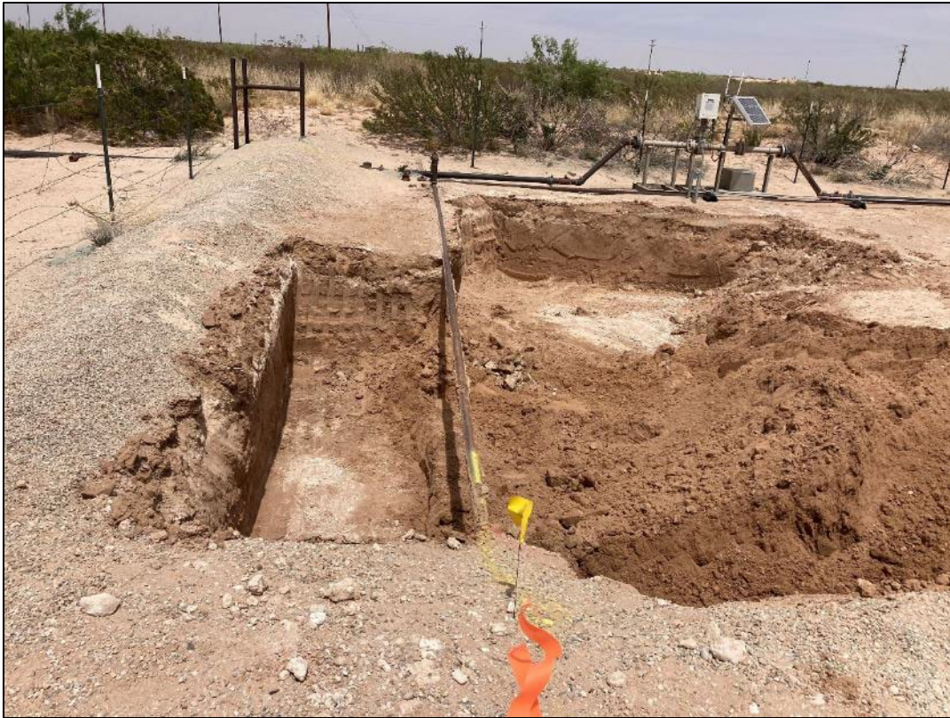
PHOTO 5: View of the excavated area facing east. 5/24/2022
