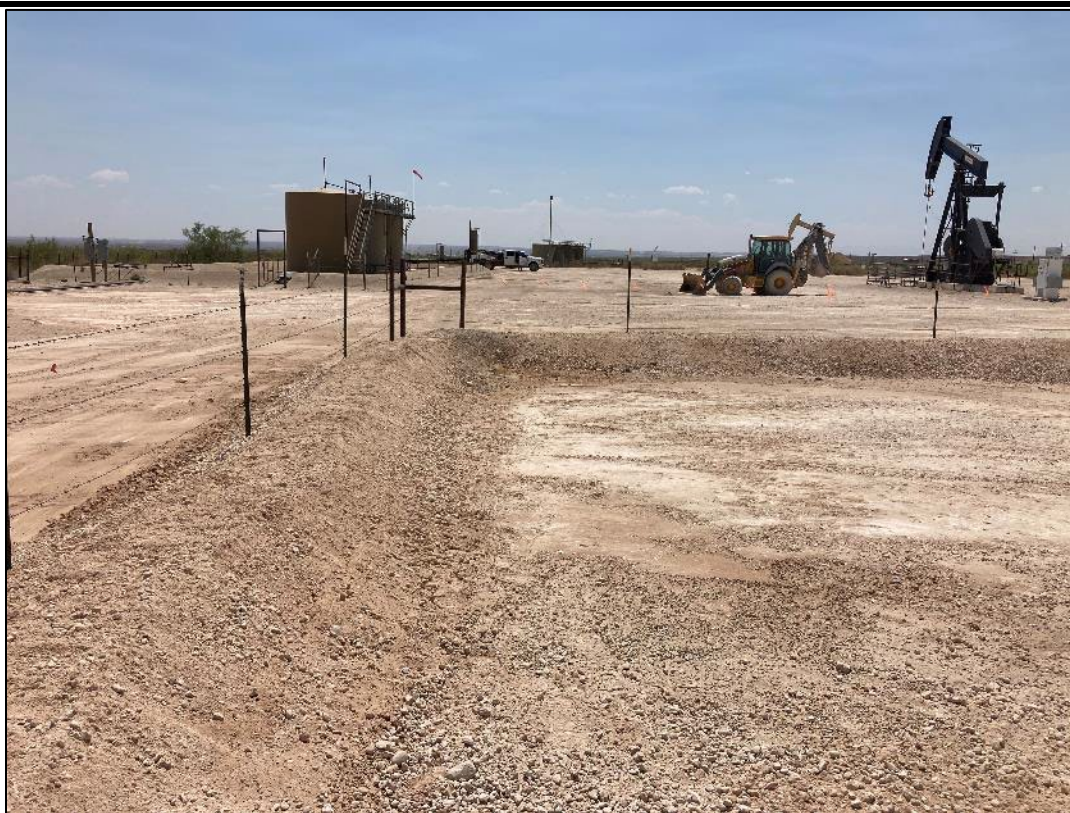
PHOTO 18: View of the remediated area facing west. 5/27/2022
