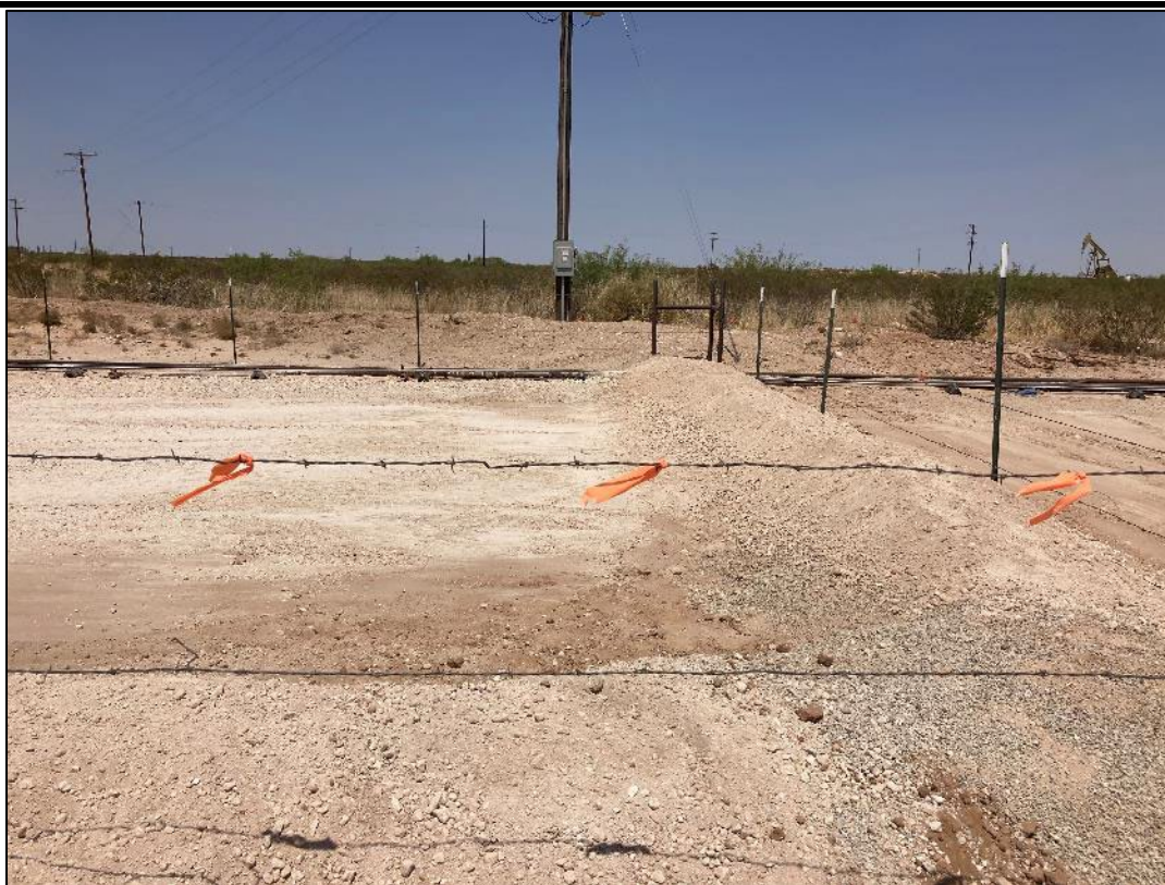
PHOTO 16: View of the remediated area facing east. 5/27/2022
