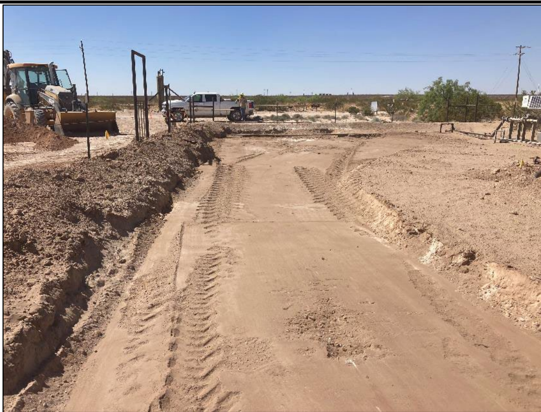
PHOTO 14: View of the area being backfilled facing north. 5/26/2022
