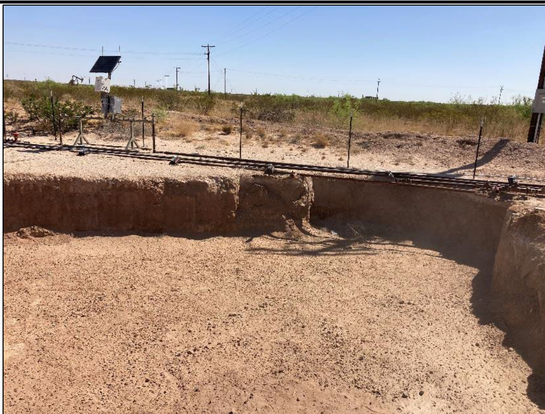
PHOTO 12: View of the excavated area facing east. 5/26/2022
