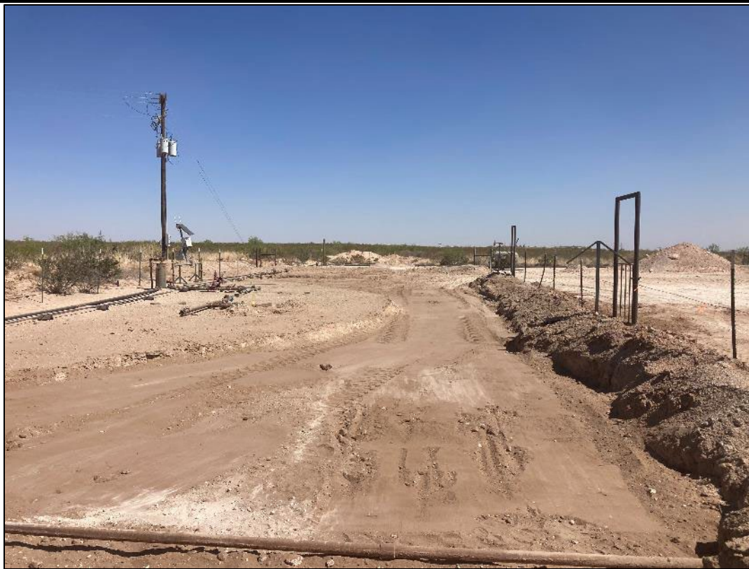
PHOTO 13: View of the area being backfilled facing south. 5/26/2022
